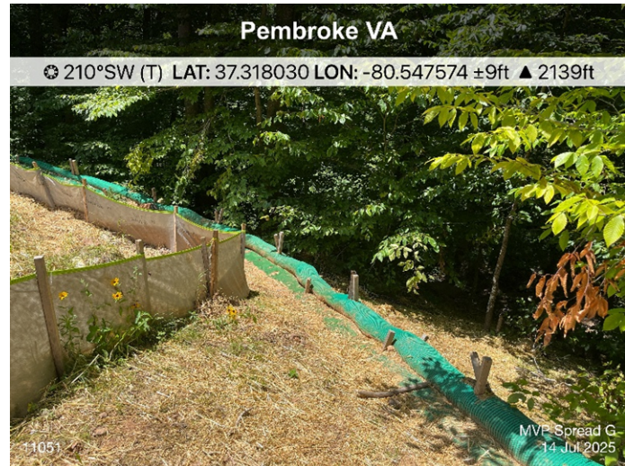
Figure 2: STA 11051, area has been repaired and stabilized.
