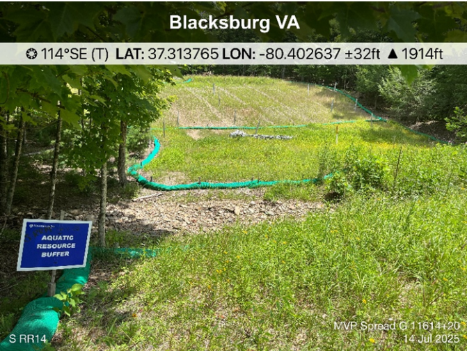
Figure 4: Designated crossing S-RR14, ESC remains in place.
