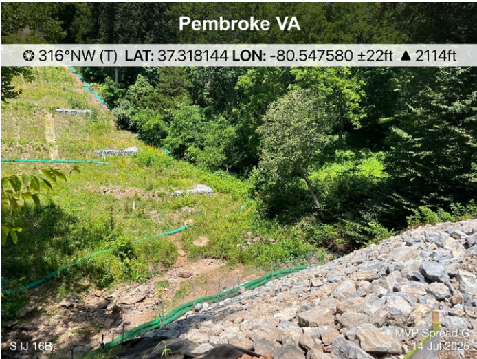
Figure 1: Designated crossing S-IJ 16B, active repairs near crossing.
