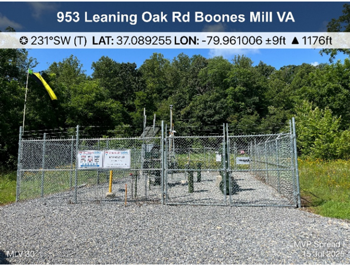
Figure 3: MLV 30, area remains stabilized.
