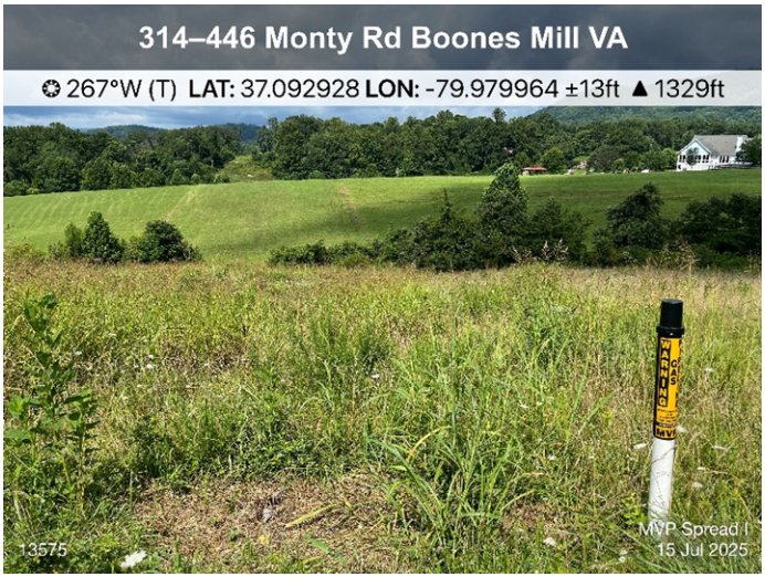
Figure 2: STA 13575, area remains stabilized.
