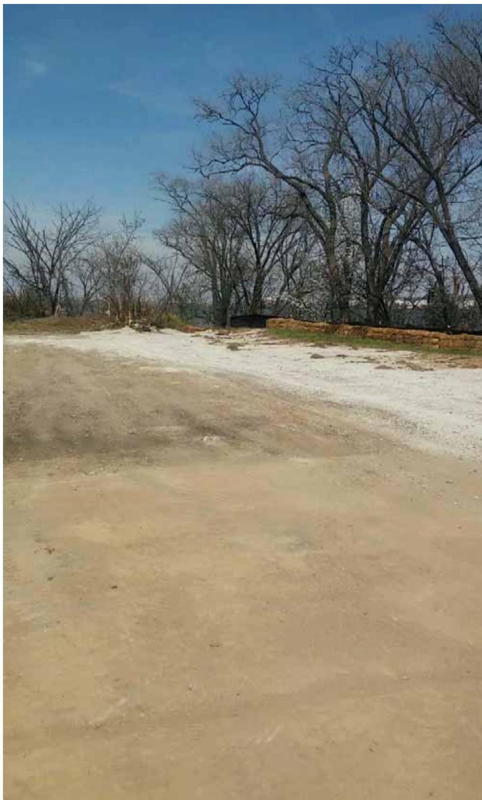
Former UST area backfilled
