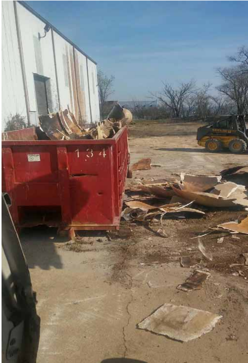
USTs, cleaned, dismantled and placed in roll off container for disposal
