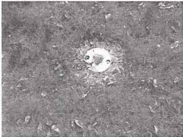
15. View of one of several monitoring wells present in the area of the diesel USTs outside the 1 Oronoco Street warehouse
