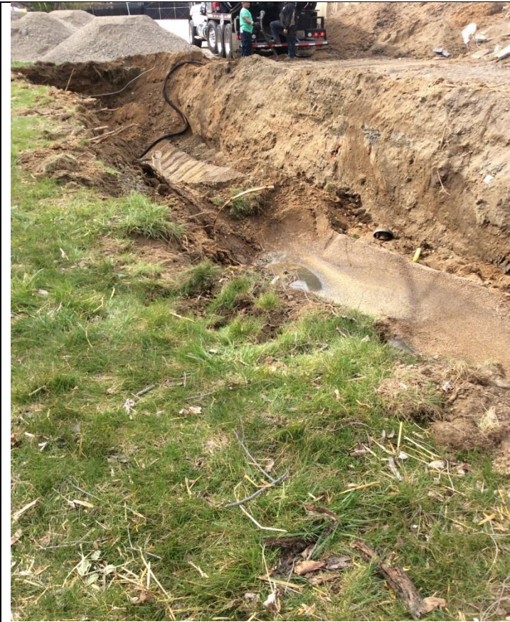
13) Pump out of water in tank trench.
