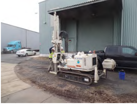
View of direct-push sampling rig used to advance test borings and install new wells (location MW-23).
