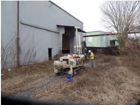
View of test boring and new well location MW-24.
