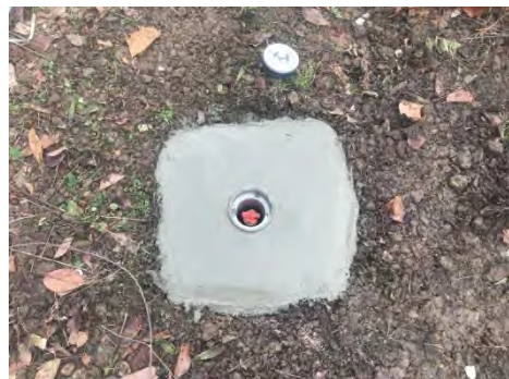
View of well completion (pad, manhole, and well cap).
