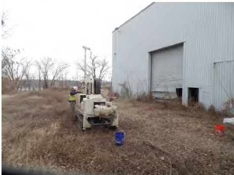
View of test boring and new well location MW-25.
