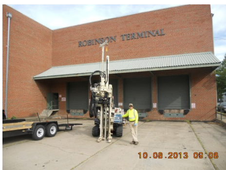
View of direct-push sampling rig during advancement of test boring ICOR-SB6.
