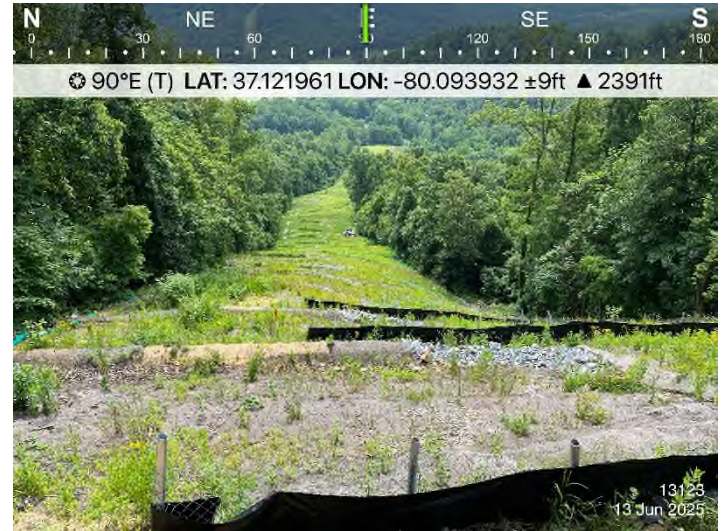
Fig. 2 STA 13123+00: Controls in place and functioning properly.
