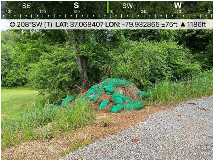
Fig. 1 MVP-FR-300: Remove damaged controls off LOD.
