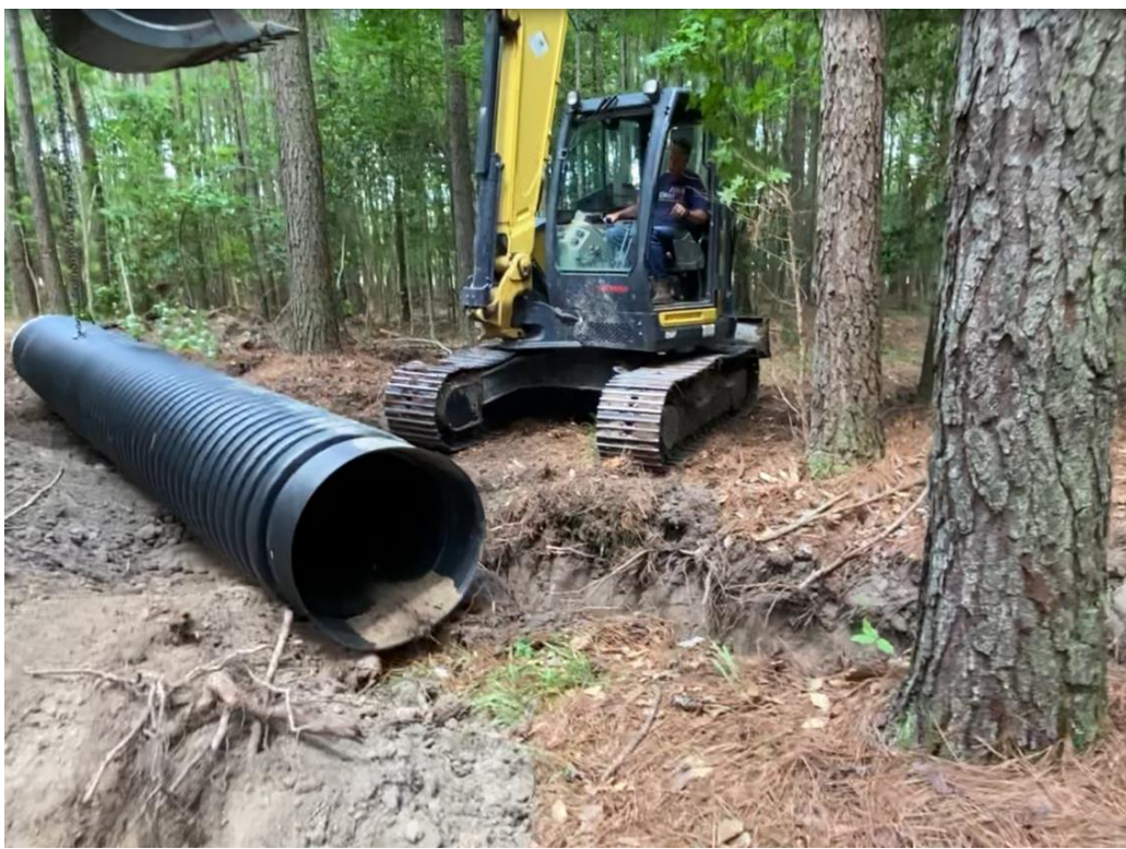
Photo 18: Culvert installation. (07/11/2024)
