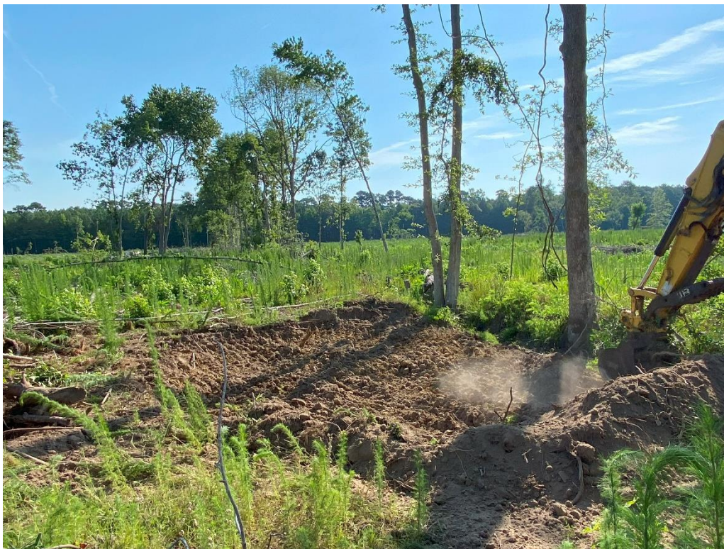
Photo 16: Wetland pool being excavated adjacent to DP 15. (07/10/2024)
