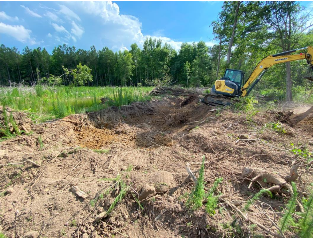
Photo 13: Excavation of a wetland pool adjacent to DP9. (07/09/2024)
