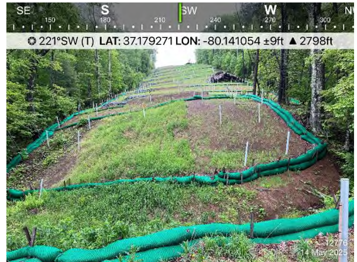
Fig. 4 STA 12776+00: Controls in place and functioning properly.
