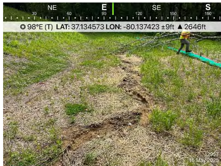
Figure 2: STA 12957+00 – Repair rilling and restabilize.
