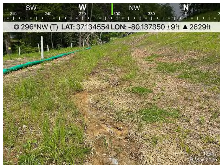
Figure 3: STA 12957+00 – Repair rilling and restabilize.
