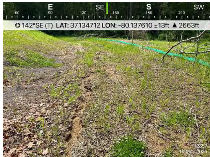
Figure 3: STA 12957+00 – Repair rilling and restabilize.
