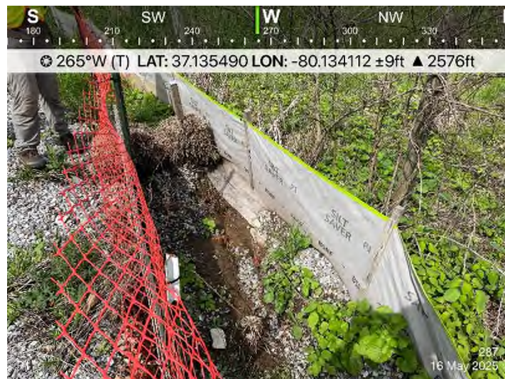
Figure 3: MVP-RO-287 – Evidence of previous gravel washing from RO-287 impacting Wetland W-IJ62. Landowner previously refused access for clean up.
