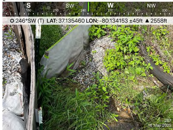
Figure 2: MVP-RO-287 – P1 SF maintenance required. Retrieve gravel.
