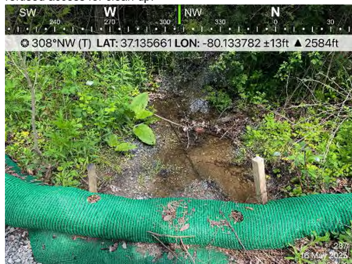
Figure 3: MVP-RO-287 – Evidence of previous gravel washing from RO-287 impacting Wetland W-IJ62. Landowner previously refused access for clean up.
