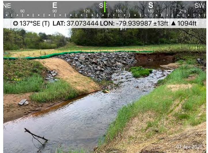
Fig. 2 Stream S-EF12: Controls in place and functioning properly.
