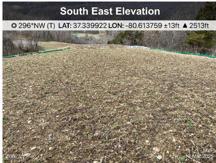
Figure 1: STA 10823, re stabilization is required on denuded areas.
