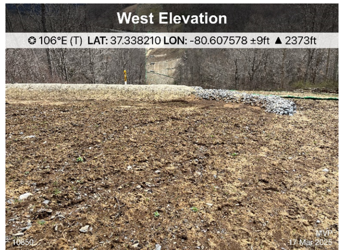
Figure 4: STA 10850, permanent waterbar requires cleanout and re stabilization.
