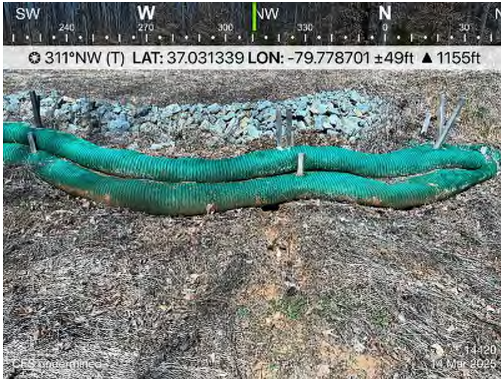
Fig. 1 STA 14420+00: CFS undermined.
