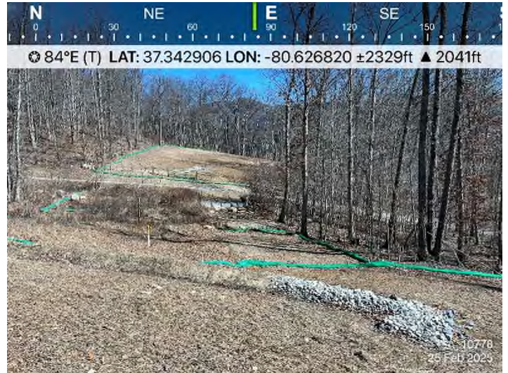
Fig. 4 STA 10778+00: Controls in place and functioning properly.
