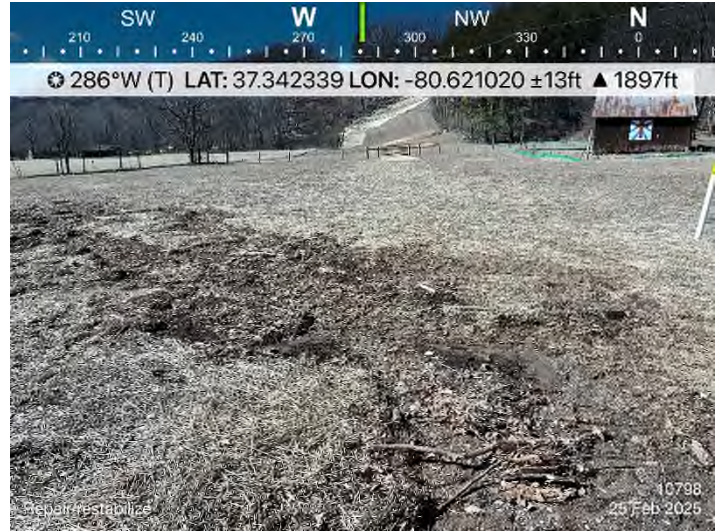
Fig. 2 STA 10798+00: Restabilize and repair rill erosion.
