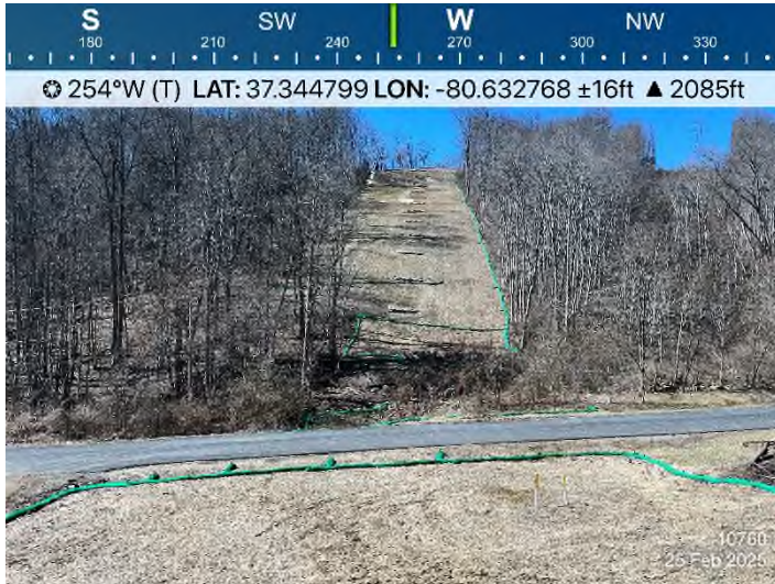
Fig. 3 STA 10760+00: Controls in place and functioning properly.
