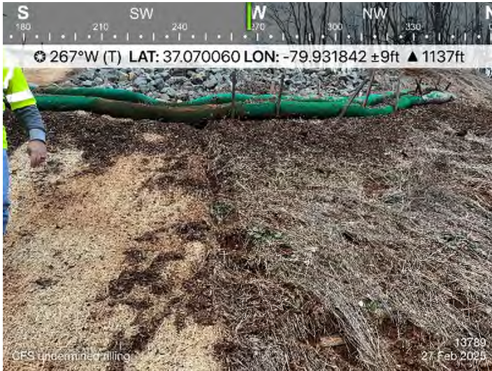
Fig. 1 STA 13789+00: CFS undermined.
