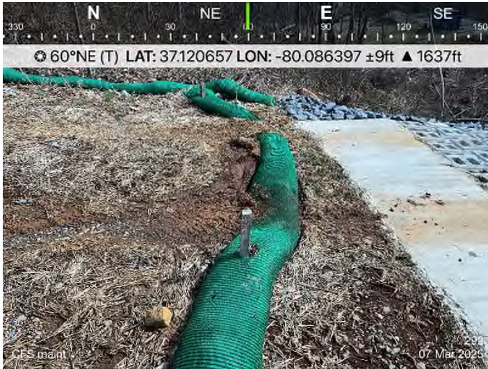
Fig. 1 MVP-FR-292: CFS maintenance required.
