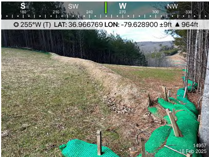
Fig. 3 STA 14957+00: Controls in place and functioning properly.
