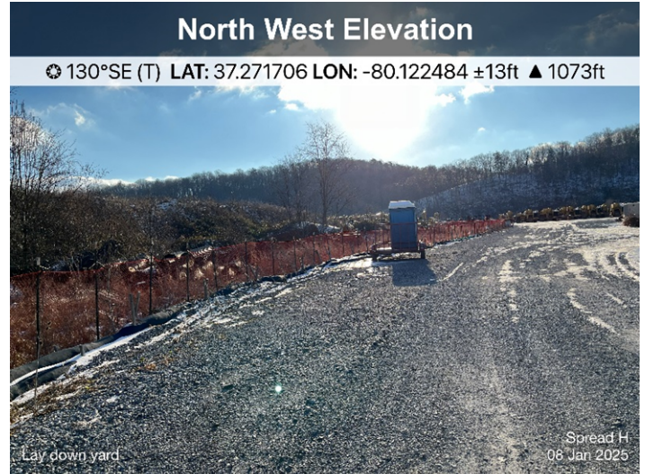
Fig. 2 LY 049, Porto johns still in place along with perimeter controls.
