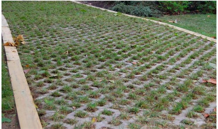
Figure D-1-2. Permeable pavement is a type of runoff reduction (RR) practice because it allows processes such as filtration and evapotranspiration to occur. This approach reduces runoff and removes a greater portion of pollutants than stormwater treatment (ST) practices that employ a permanent pool – such as wet ponds, wet swales, and constructed wetlands – because such practices simply provide storage and treatment before discharge. Photo: CBP.
