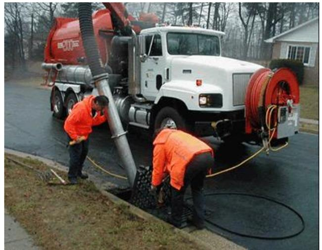
Figure D-10-1. Storm Drain Cleaning in Anne Arundel County. Work is completed on a rotating basis using a vacator (vacuum) truck to reduce sediment traveling to the Bay. Source: Anne Arundel County, Department of Public Works. [https://www.aacounty.org/departments/public-works/highways/road-maintenance/Drainage\\_Maintenance/storm-drain-cleaning](https://www.aacounty.org/departments/public-works/highways/road-maintenance/Drainage_Maintenance/storm-drain-cleaning)
