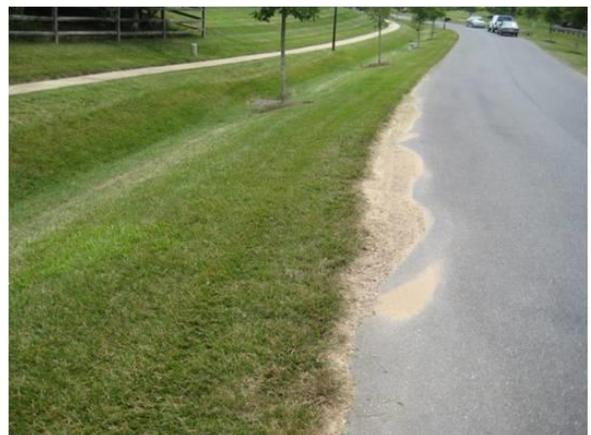
Figure D-14-2. An urban filter strip hard at work. Source: Chesapeake Stormwater Network.
