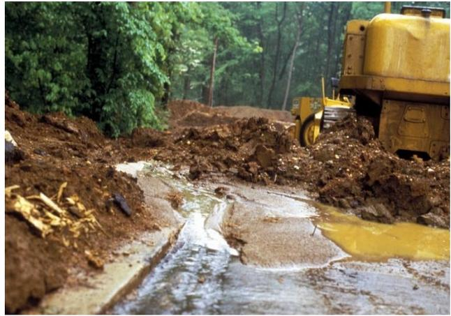
Figure D-3-1. Sediment running off a construction site. Source: Chesapeake Bay Program.
