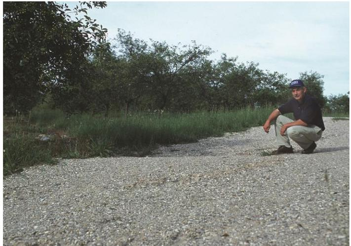
Figure D-4-1. "Resource Conservationist shows a water bar erosion control practice on a gravel road adjacent to an orchard. Grand Traverse County, Michigan." Source: USDA NRCS.
