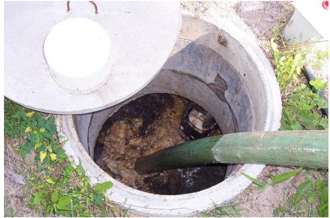
Figure S-1-1. Pumping sludge out of a septic tank, a routine part of septic system maintenance. Source: MCPA Flickr. (<https://flic.kr/p/UScorM>).
