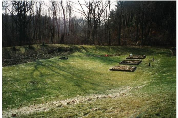
Figure D-13-1. Small dry detention basin near Harvest Circle, Village of Oregon, Wisconsin, USA. Water ponds in this area during heavy rainstorms, and slowly drains out through a pipe in the berm on the far side of the basin. Source: Aaron Volkening, Flickr (<https://flic.kr/p/dreYBM>).
