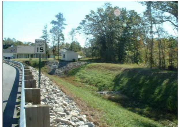
Figure D-13-2. Dry detention basin. Source: Simpson and Weammert-Lane Report (p. 201).
