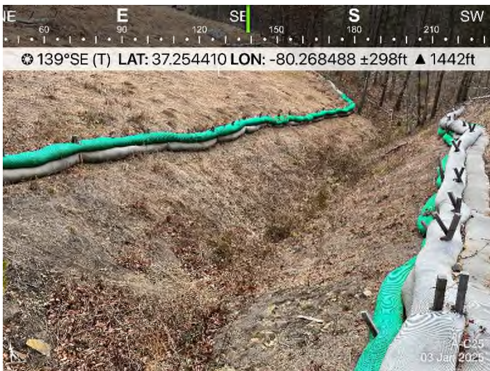
Fig. 3 Stream S-C25: Controls in place and functioning properly.
