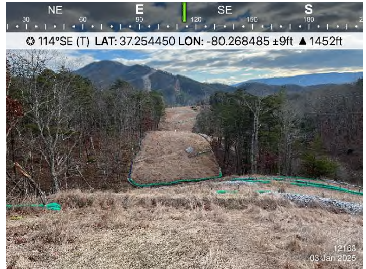
Fig. 2 STA 12163+00: Controls in place and functioning properly.
