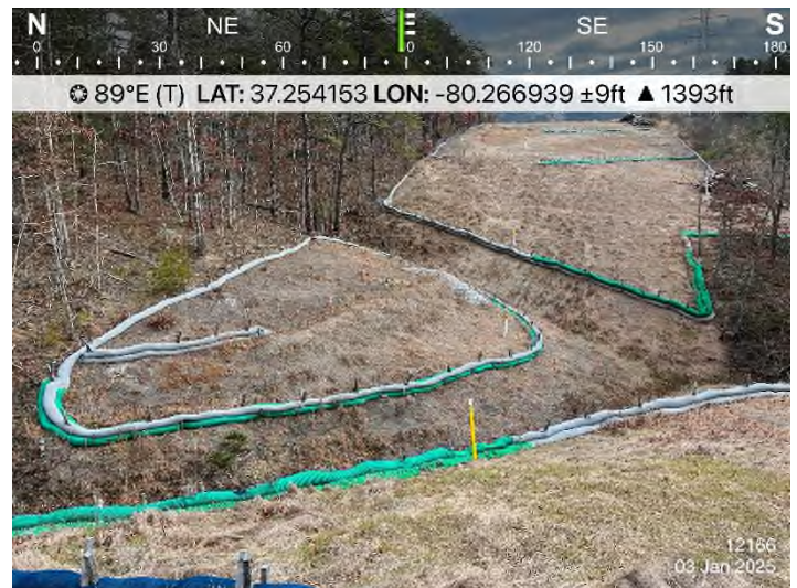
Fig. 4 STA 12166+00: Controls in place and functioning properly.
