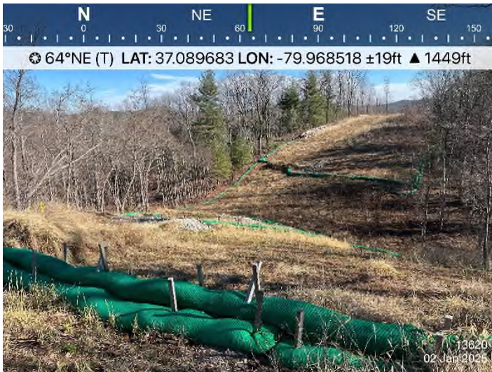
Fig. 3 STA 13620+00: Controls in place and functioning properly.
