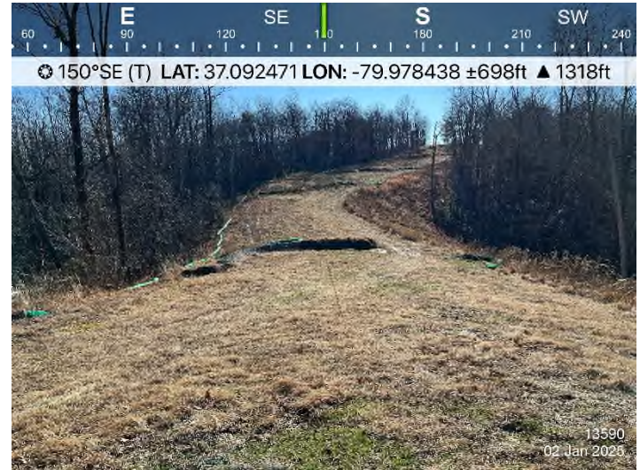
Fig. 2 STA 13590+00: Controls in place and functioning properly.
