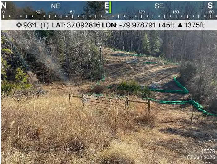
Fig. 1 STA 13579+00: Controls in place and functioning properly.
