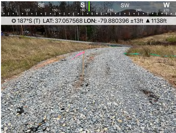
Fig. 3 MVP-MLV-AR-31: Staked for BMP installation.
