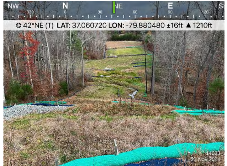
Fig. 2 STA 14033+00: Controls in place and functioning properly.
