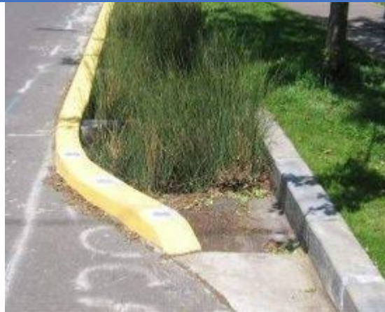
Figure P-FIL-05 B-3 Stormwater curb extensions
