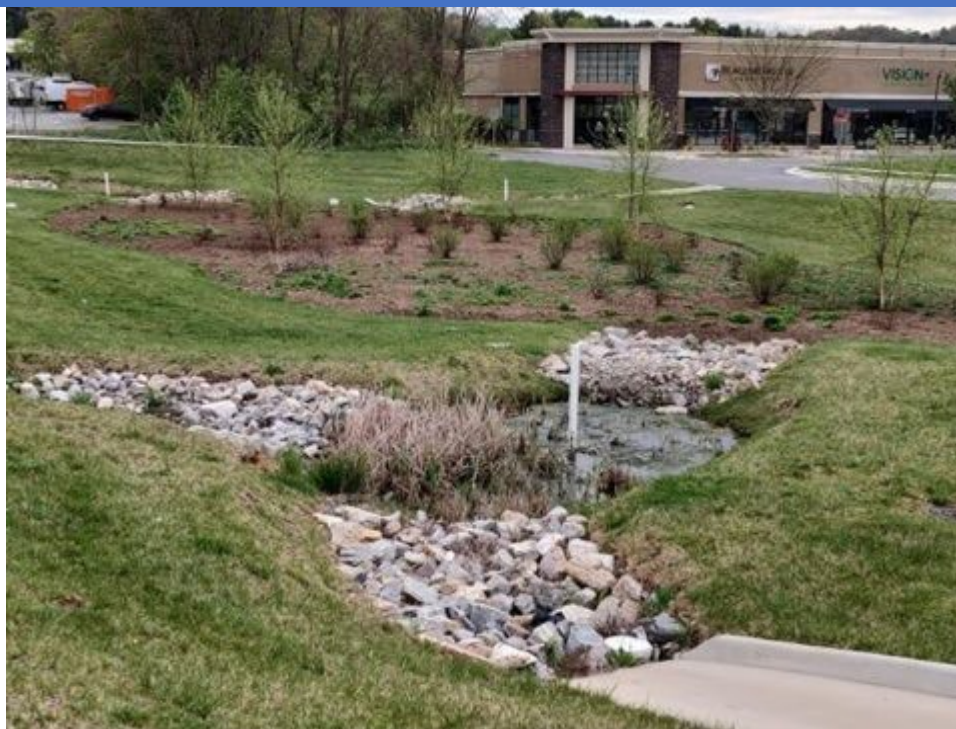
Figure P-FIL-05-3 Image of bioretention cell receiving stormwater runoff from multiple input points (3) in a mixed-use development in Blacksburg, VA
