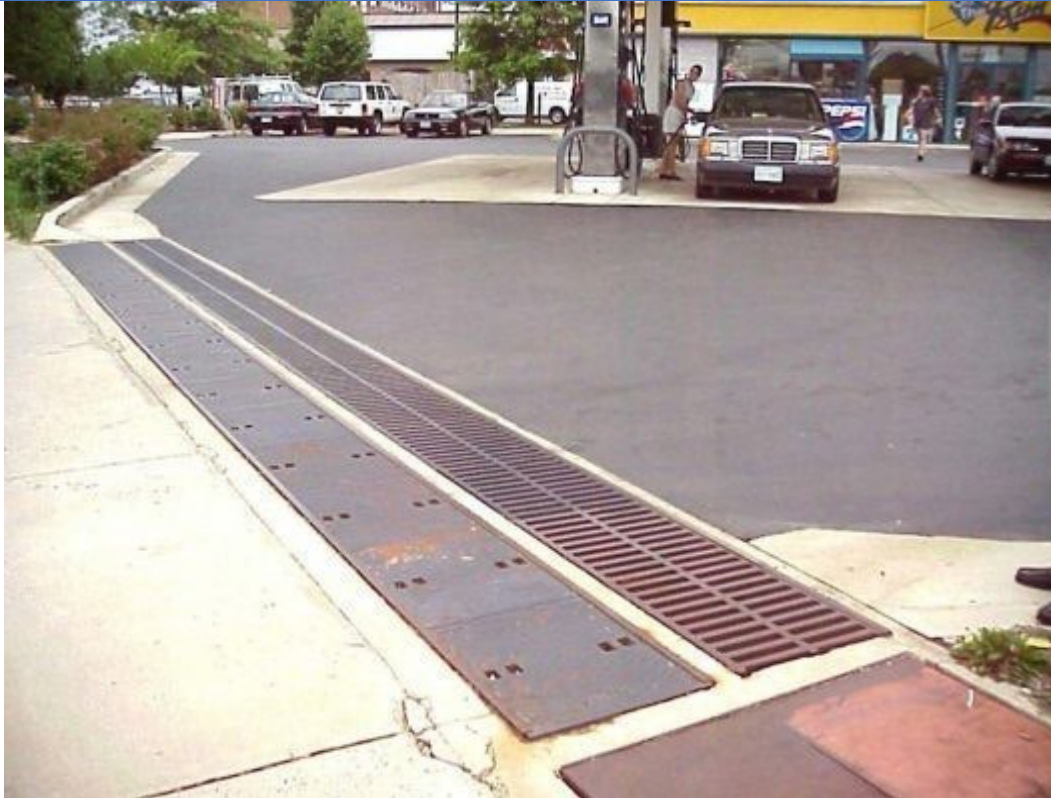
Figure P-FIL-06-3 Perimeter Sand Filter
