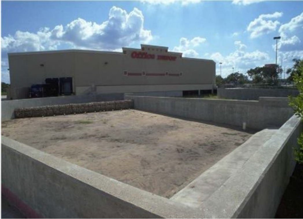
Figure P-FIL-06-2 Austin Surface Sand Filter
