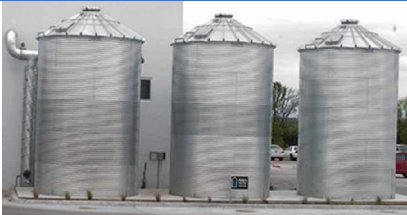
Figure P-BAS-04-6 Galvanized Steel Tanks
