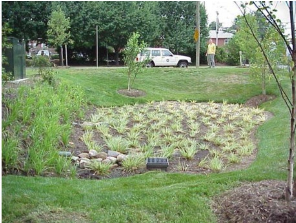
Figure P-FIL-05-1 Image of typical bioretention practice
