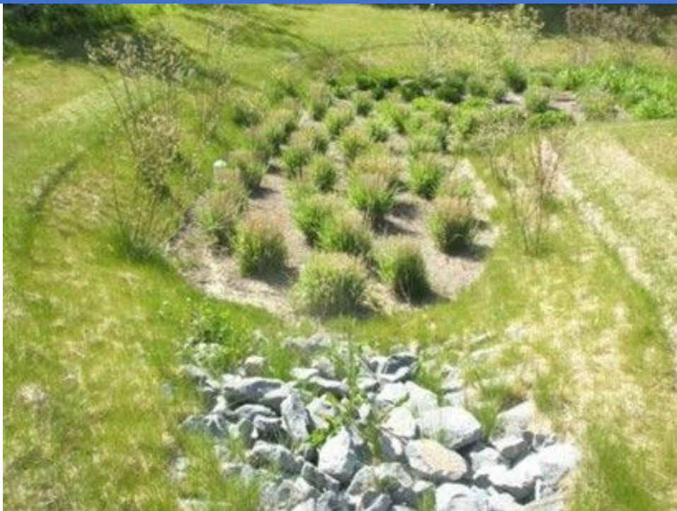
Figure P-FIL-05-2 Image of typical bioretention practice
