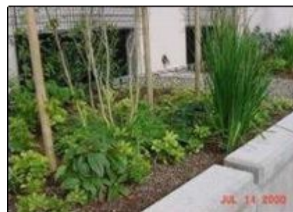
Stormwater Curb Extensions
