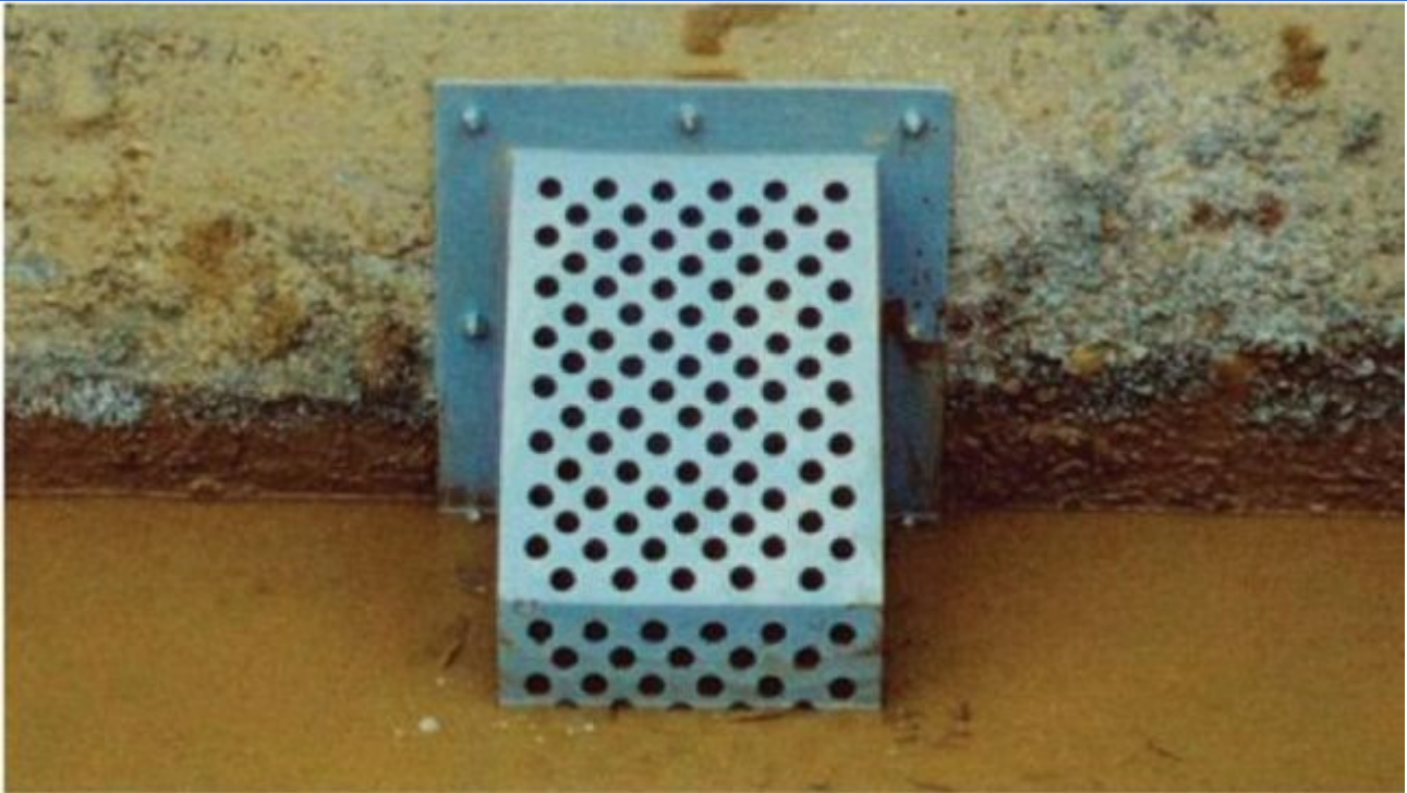
Figure P-SUP-06-5 Manufactured Coarse Solids Screen
