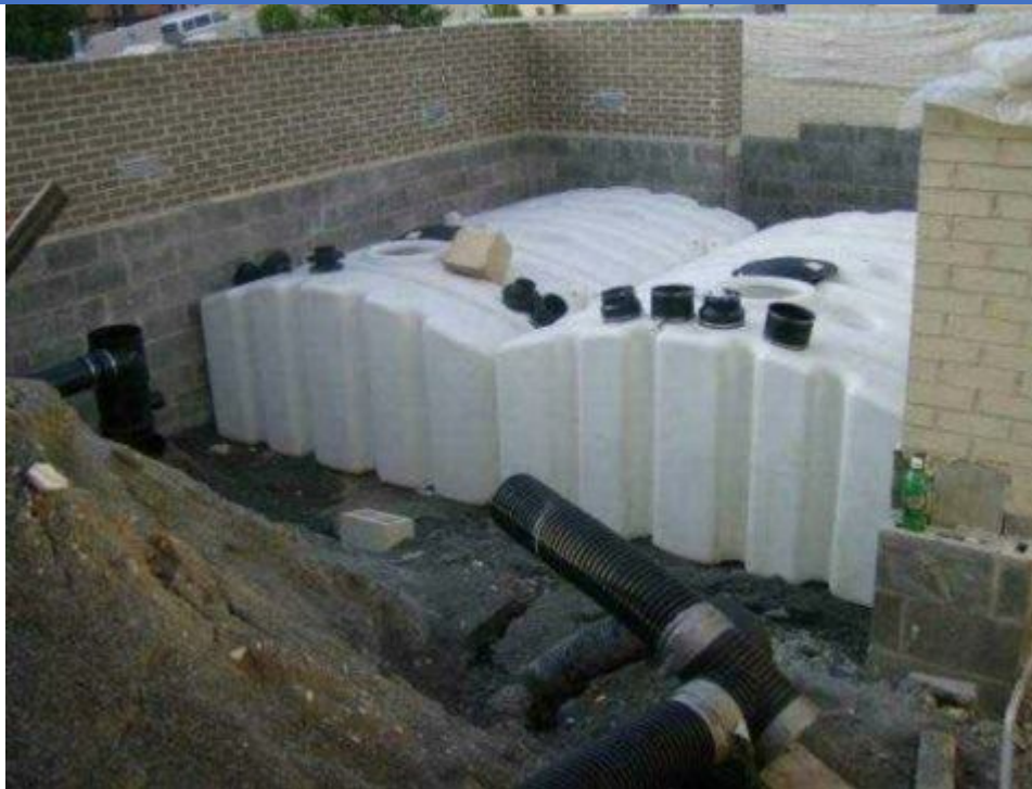
Figure P-BAS-04-5 Example of two Polyethylene Cisterns
