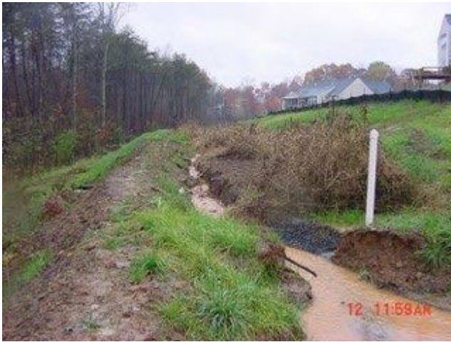
Dry swale in operation too early in construction sequence. Photo Credit: Hirschman Water & Environment, LLC
