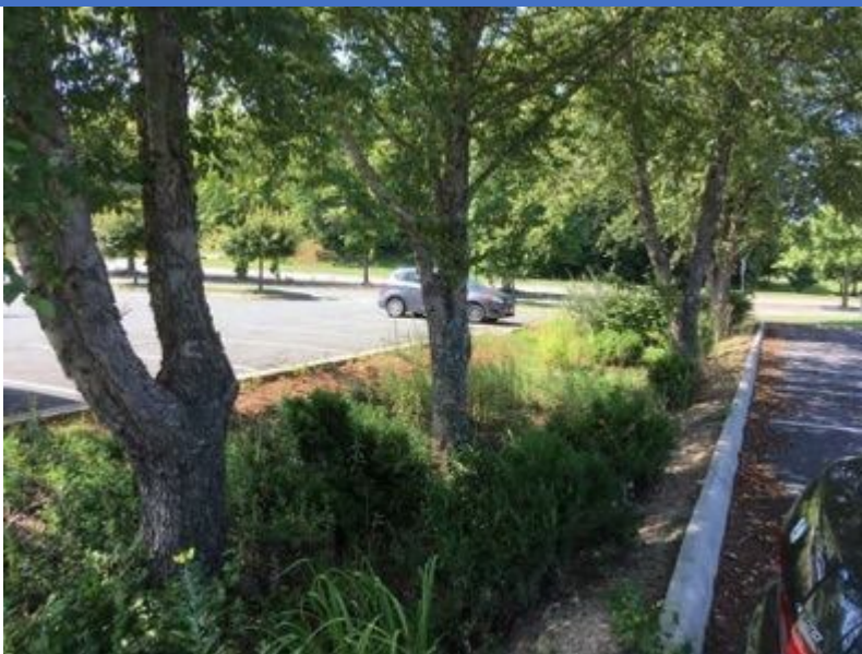
Figure P-FIL-05-12 An older bioretention area with mature tree growth and shaded areas.
