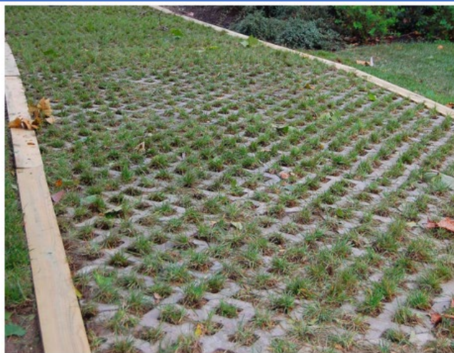
Figure P-FIL-03-1 Types of Permeable Pavement: (clockwise from upper left): Concrete Grid Pavers (Chesapeake Stormwater Network); Pervious Concrete (perviouspavement.org), Permeable Interlocking Concrete Pavers (UC Davis), Porous Asphalt (UC Davis)
