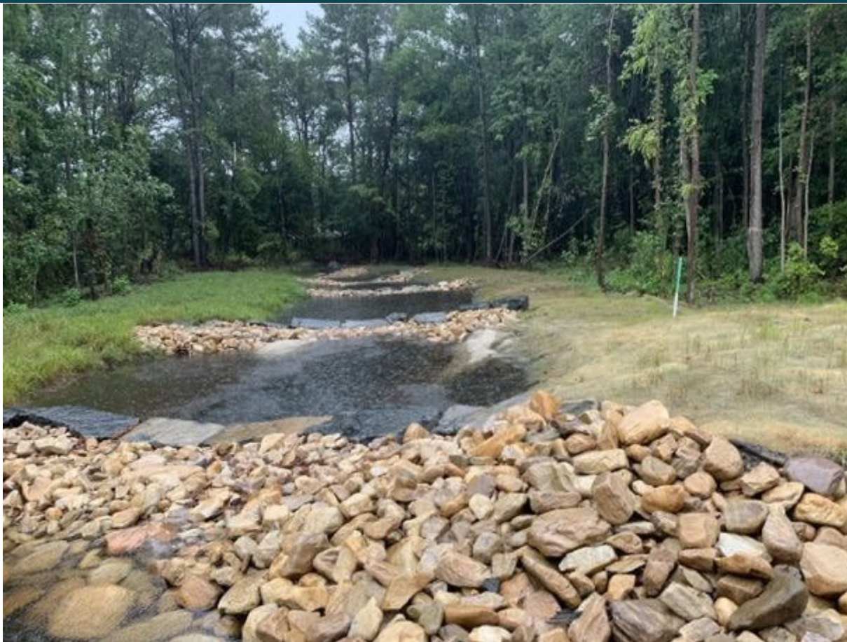
Figure P-CNV-04-1 Newly constructed regenerative stormwater conveyance Chesterfield County Complex
