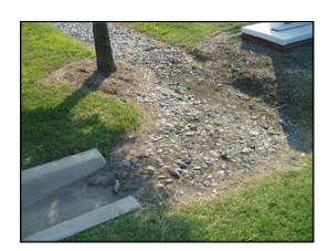
Too much mulch and grass clippings, and overgrowth of grass which over time would lead to thick mat of weeds over gravel
