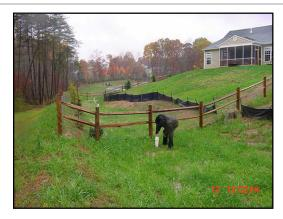
Silt fence is used in this picture to keep sediment out of the P-CNV-02 Dry Swale while the swale stabilizes.
