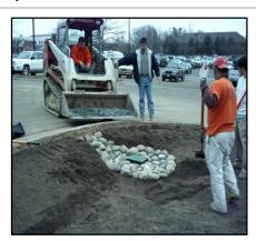
Inlet is temporarily blocked during installation of this P-FIL-05 Bioretention.
