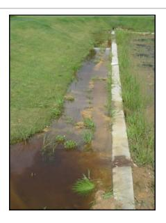
Level spreader showing signs of standing water, short-circuiting, and sediment/debris
