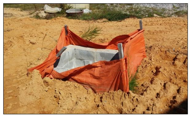
Improper installation of silt fence inlet protection
