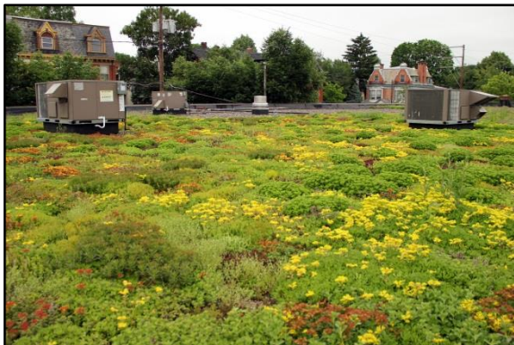
Figure 16: Extensive green roof
