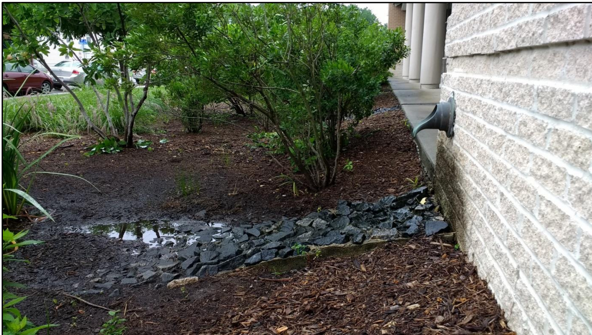
Figure 15: Rooftop disconnection to rain garden
