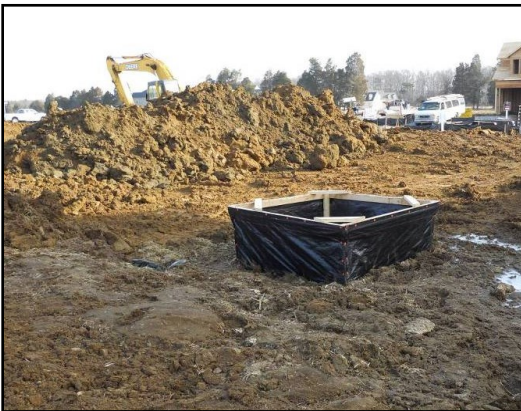
Silt fence drop inlet protection
