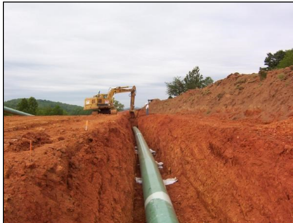
Backfilling a utility trench
