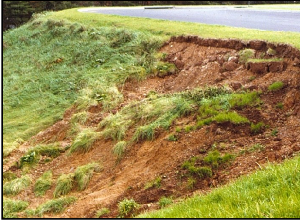
Slope failure from a water seep
