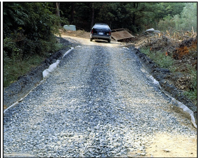
Temporary stone construction entrance (C-SCM-02)
