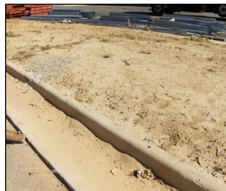
Figure 1: Sedimentation resulting from missing Construction BMPs.
