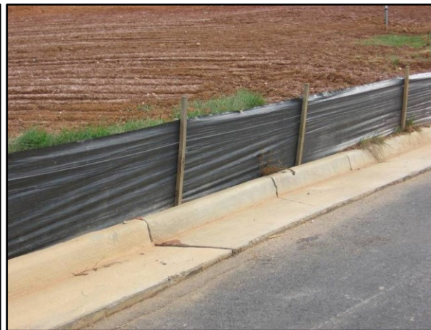
Silt fence with wooden stakes (C-PCM-04)
