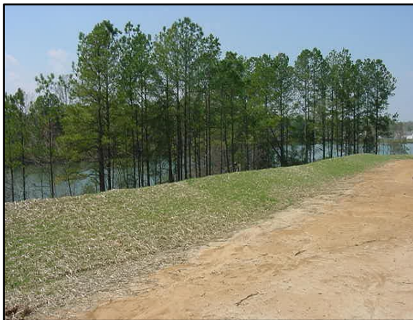
Stabilized perimeter diversion dike (C-ECM-04)
