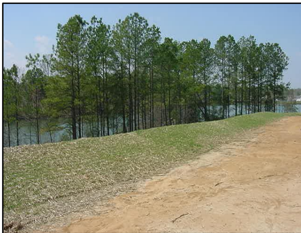
Stabilized perimeter diversion dike (C-ECM-04)
