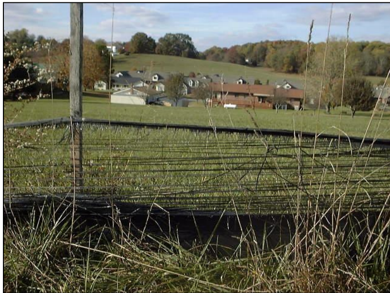
Silt fence must be removed at end of project.
