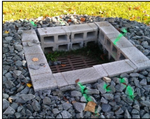
Block and gravel drop inlet sediment filter
