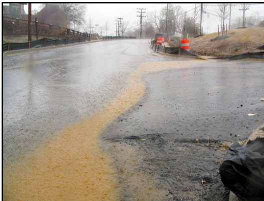
Figures 12 and 13: Construction site erosion and runoff
