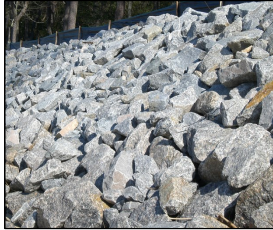
Riprap installed to prevent further slope failure
