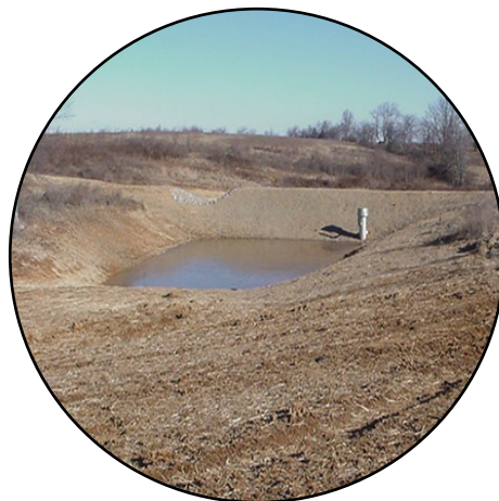
Sediment Basin Drainage areas \geq 3 acres
