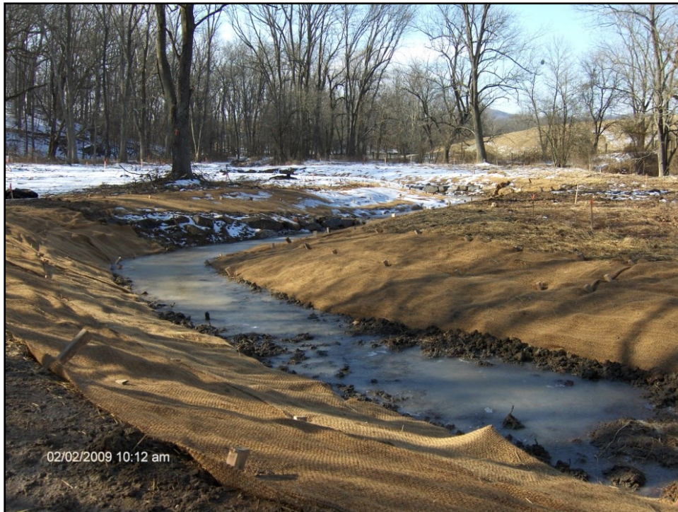
Vegetative streambank stabilization
