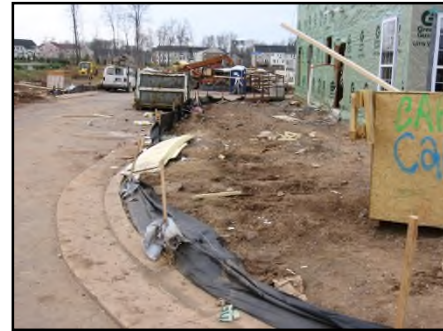
Figure 2: Trash around construction site – pollution prevention measures not in place
