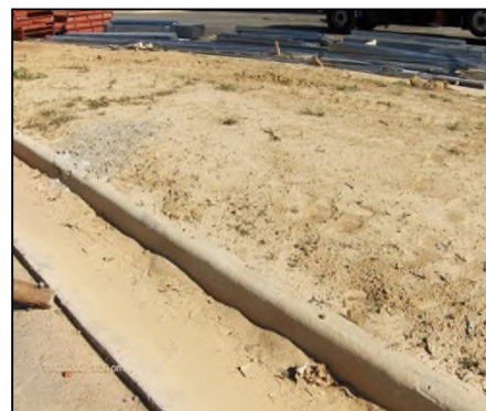
Figure 1: Sedimentation resulting from missing Construction BMPs.
