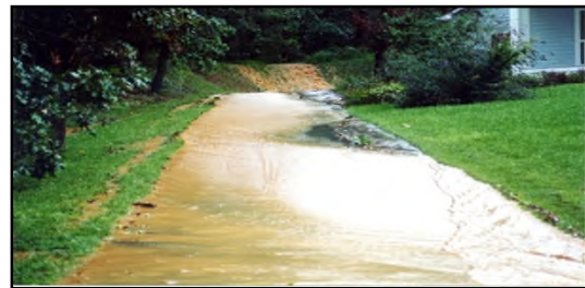
Figure 3: Flooding of downstream properties from inadequate post-construction stormwater management
