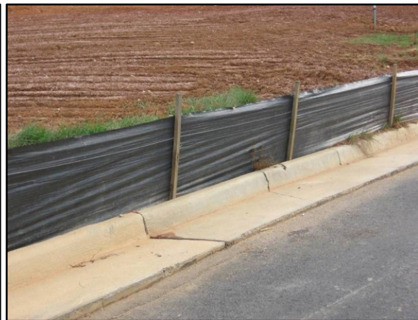
Silt fence with wooden stakes (C-PCM-04)
