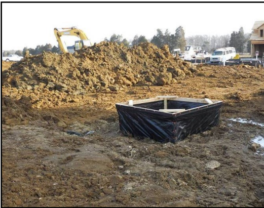
Silt fence drop inlet protection
