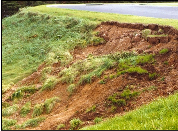
Slope failure from a water seep
