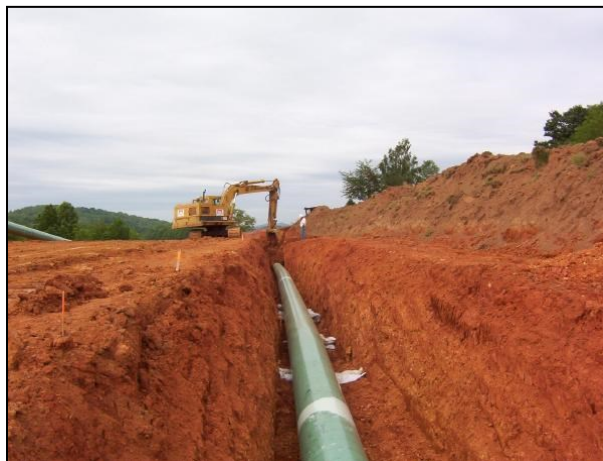
Backfilling a utility trench
