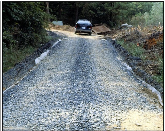
Temporary stone construction entrance (C-SCM-02)
