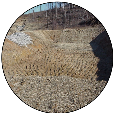
Sediment Trap Drainage areas < 3 acres
