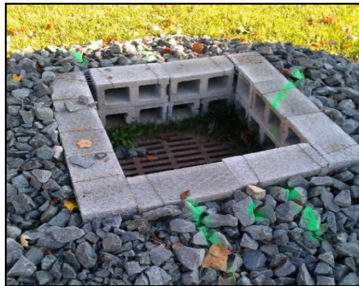
Block and gravel drop inlet sediment filter
