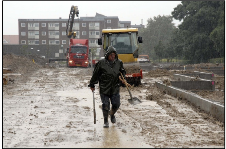
Figure 7: Sediment-laden water and raindrop impact are slowly sealing the soil across this construction site.
