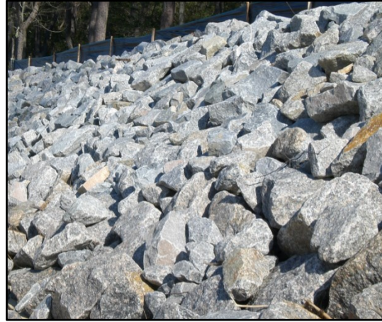
Riprap installed to prevent further slope failure
