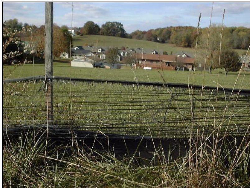
Frayed and weathered silt fence not removed at end of project.
