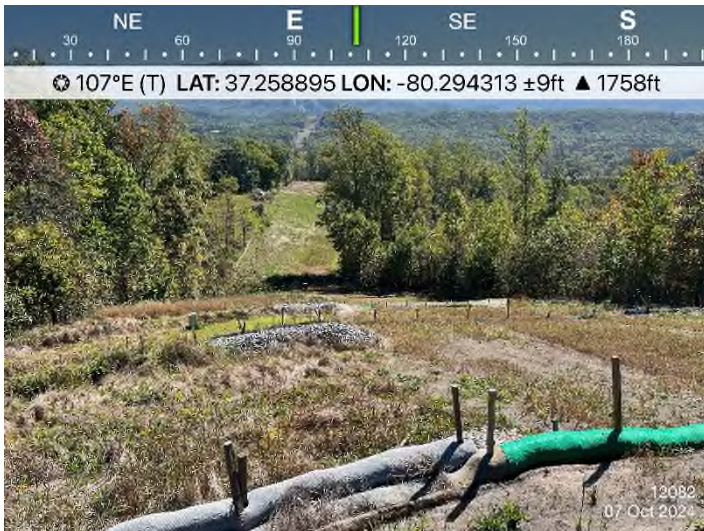
Fig. 3 STA 12082+00: Controls in place and functioning properly.
