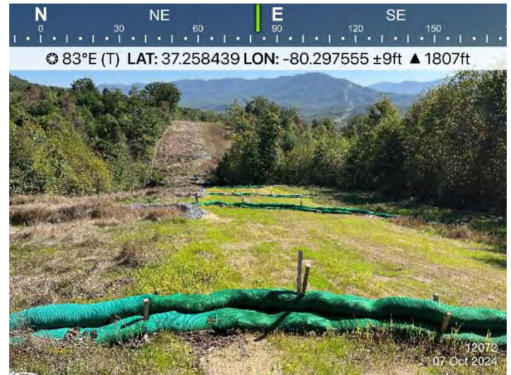
Fig. 4 STA 12072+00: Controls in place and functioning properly.
