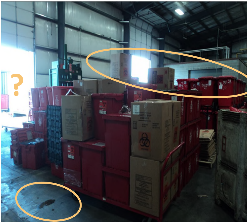
Staging area for RMW; boxes are stacked too high (higher than 6 ft); note wet area on the floor
