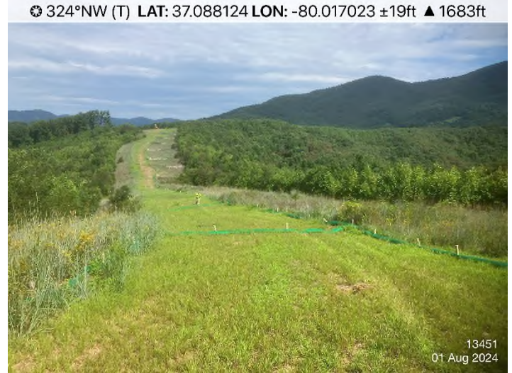
Fig. 2 STA 13451+00: Controls in place and functioning properly.
