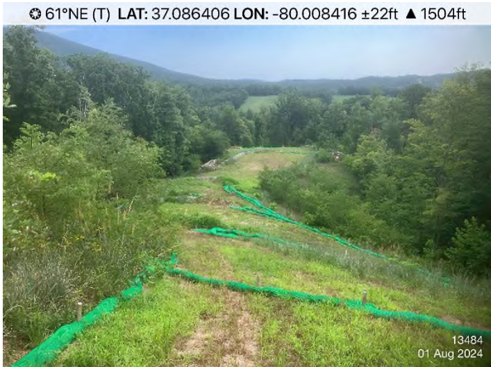
Fig. 3 STA 13484+00: Controls in place and functioning properly.
