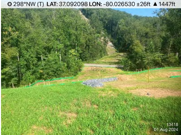
Fig. 1 STA 13418+00: Controls in place and functioning properly.
