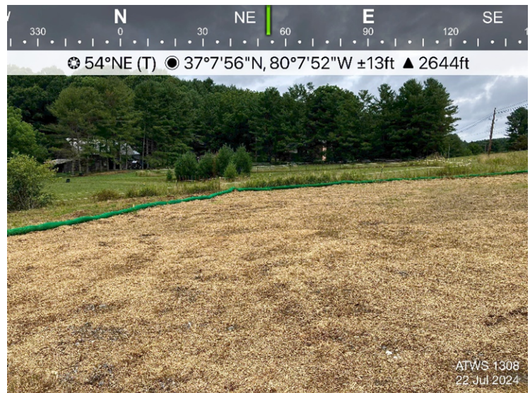
Figure 4: ATWS 1308, stabilization has been applied and ESC is in place.
