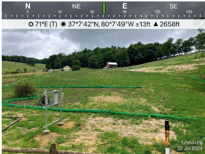
Figure 1: Sta 12994+26, ESC's devices and stabilization are in place.
