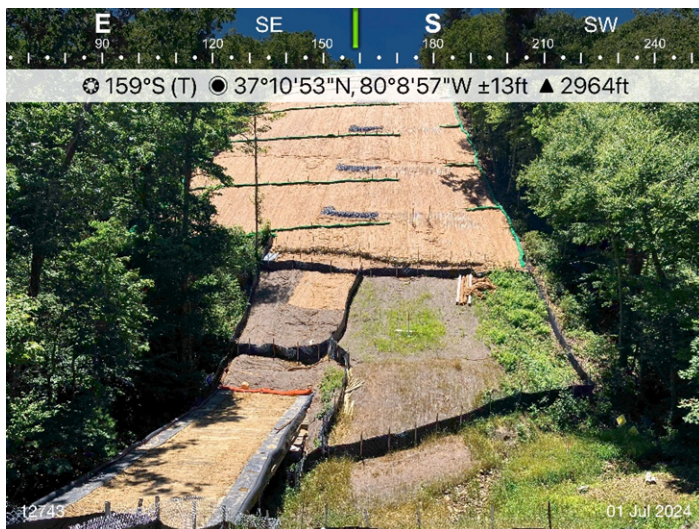
Figure 3: Designated crossing S-EF 34ESC's devices and permanent waterbars are in place.
