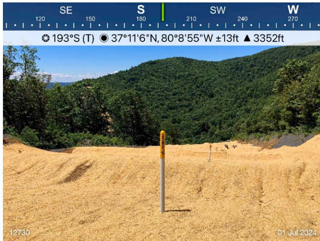
Figure 1: Sta 12730, ESC's devices in place.
