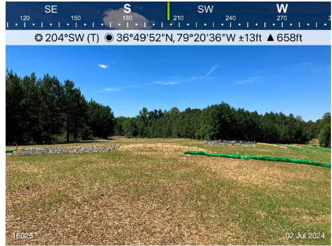
Figure 2: Sta 16025, ESC and permanent water bars are in place.
