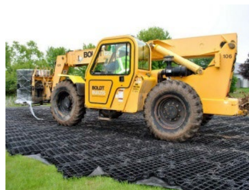
Rubber Equipment Pads for Wetland Crossing Source: Presto Geosystems 2016
