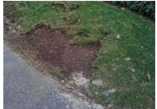
Unclean and Poor Sod Installation
