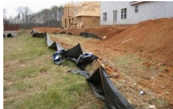
Silt Fence Failure
