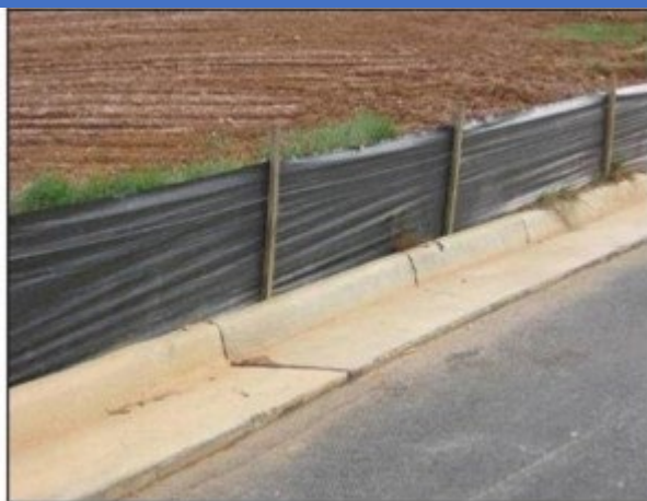
Figure 5-10 Silt Fence Perimeter Control
