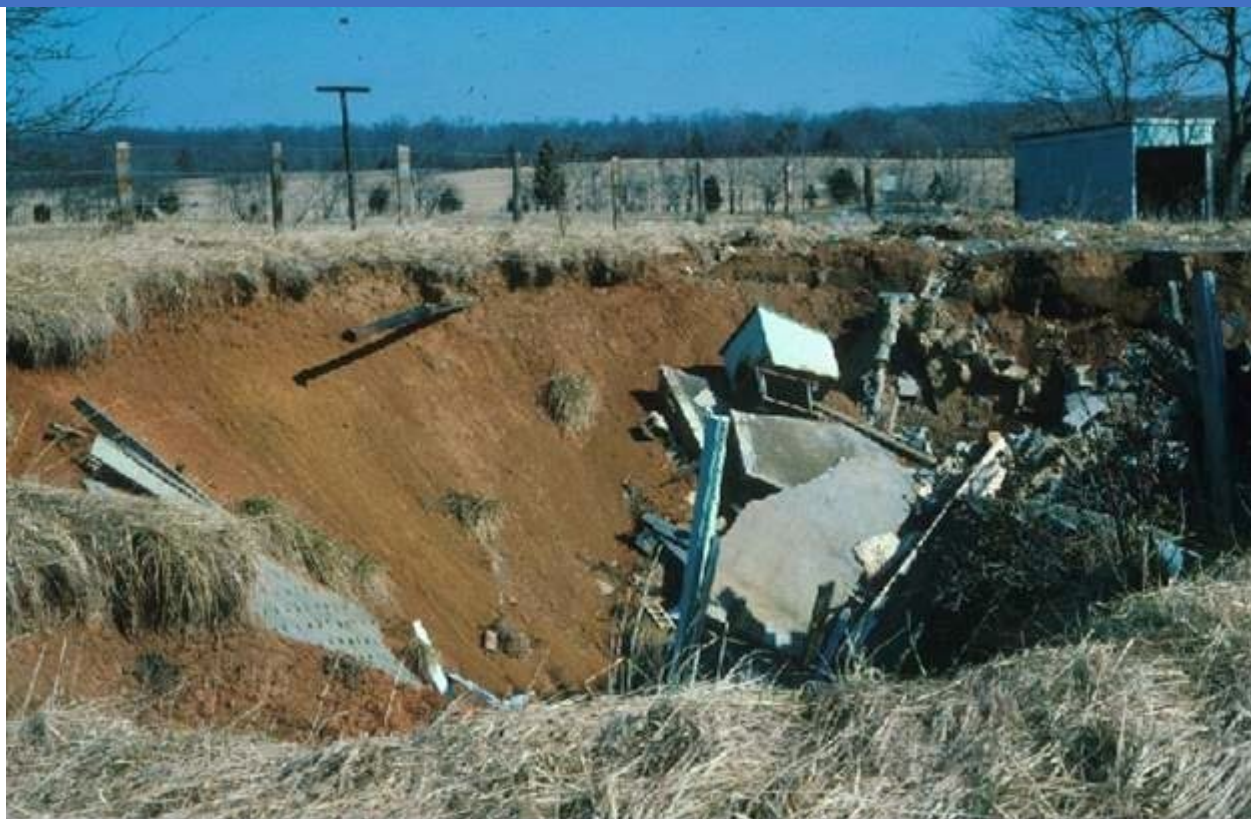
Figure E-11 A house swallowed by a sinkhole near Berryville, Virginia in 1992, believed to be induced by nearby well drilling
