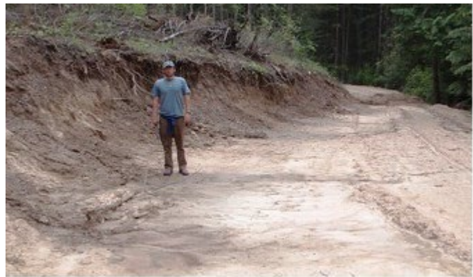
Surface Roughening Ignored on Side Slopes of Access Road
