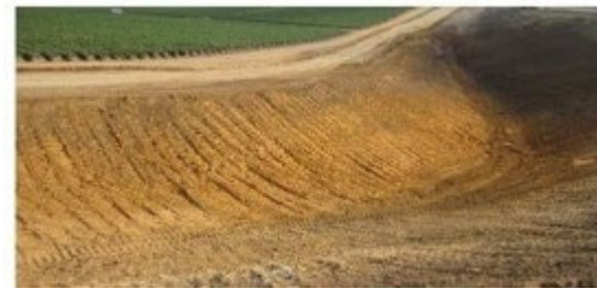
Effective and Proper Surface Roughening Source: USEPA 2021
