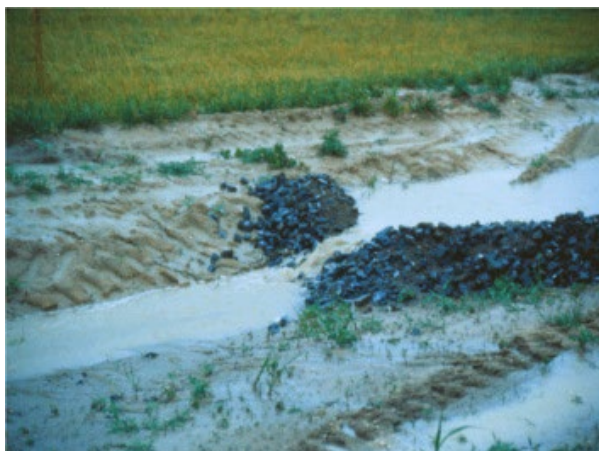
Improperly Installed or Maintained Rock Check Dam Failing Under Wet Conditions
