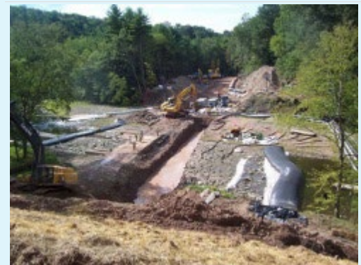
Active Dam and Pump Bypass Stream
