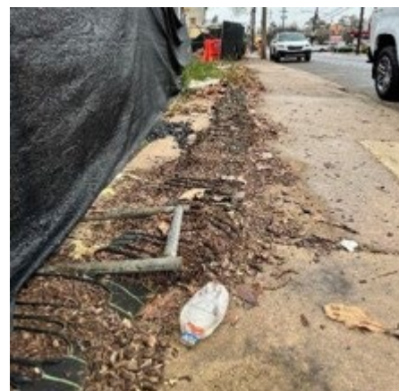
Improperly Maintained Compost Filter Sock
