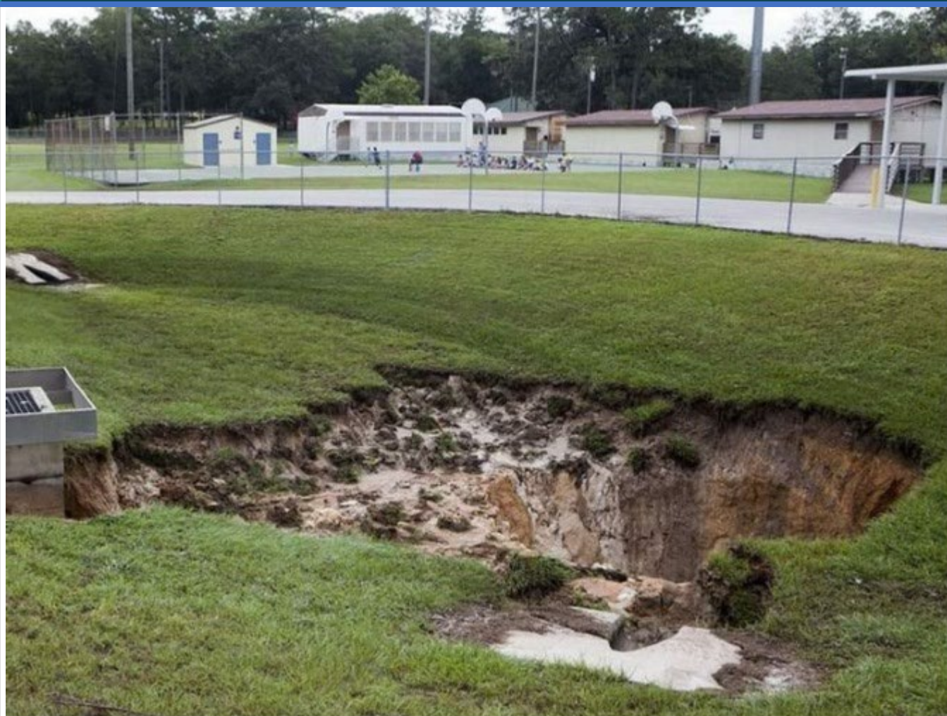
Figure 10-5 BMP Sinkhole Collapse
