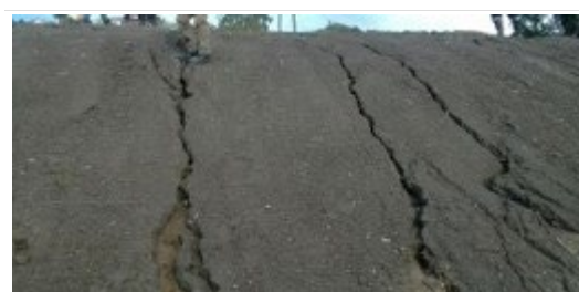
Topsoiling Application Failed Source: Environment Canterbury Regional Council 2017
