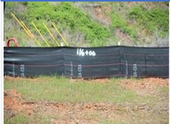
Figure 6-28 Silt Fence Perimeter Control Practice
