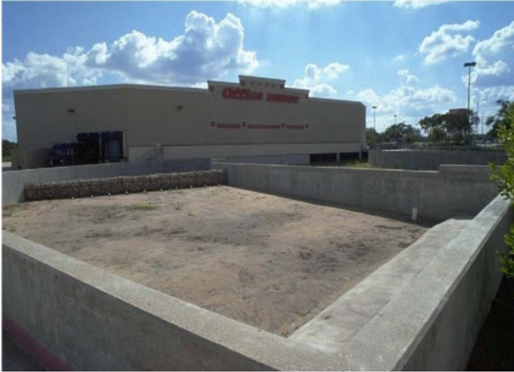
Figure P-FIL-06-2 Austin Surface Sand Filter
