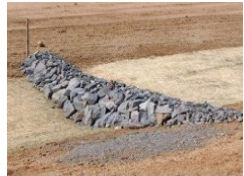
A Rock Check Dam Under Dry Conditions Source: Earth Tek, Inc. 2014.
