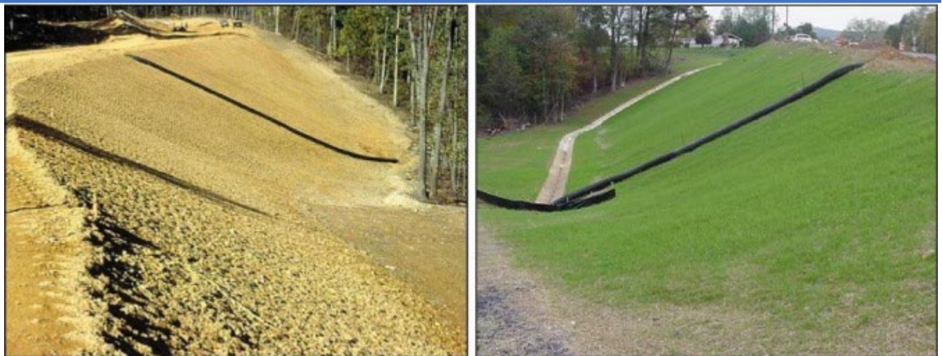
Figure 5-15 Slope Stabilization with Slope Drains to Reduce Concentrated Runoff
