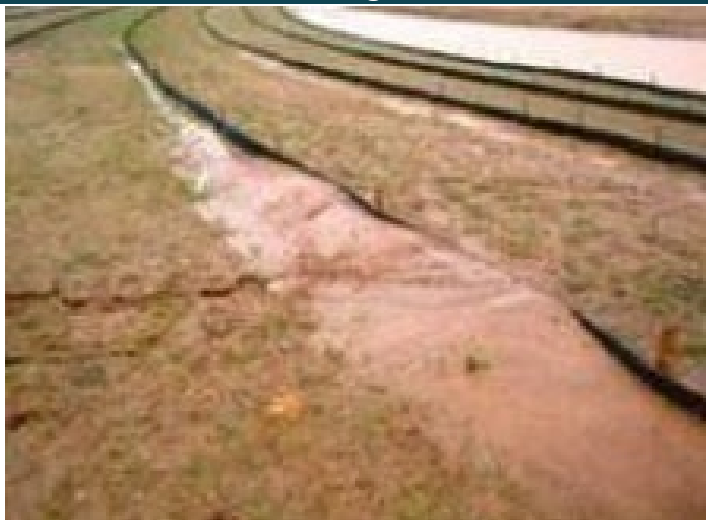
Figure C-ECM-03-1 Slope Interruption Device Accumulating Sediment
