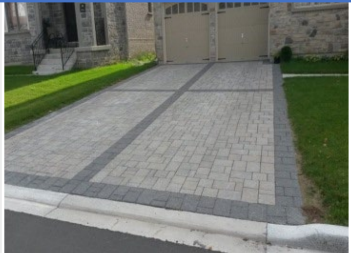
Figure 6-12 Permeable Pavers Replace Concrete or Asphalt for Residential Driveways
