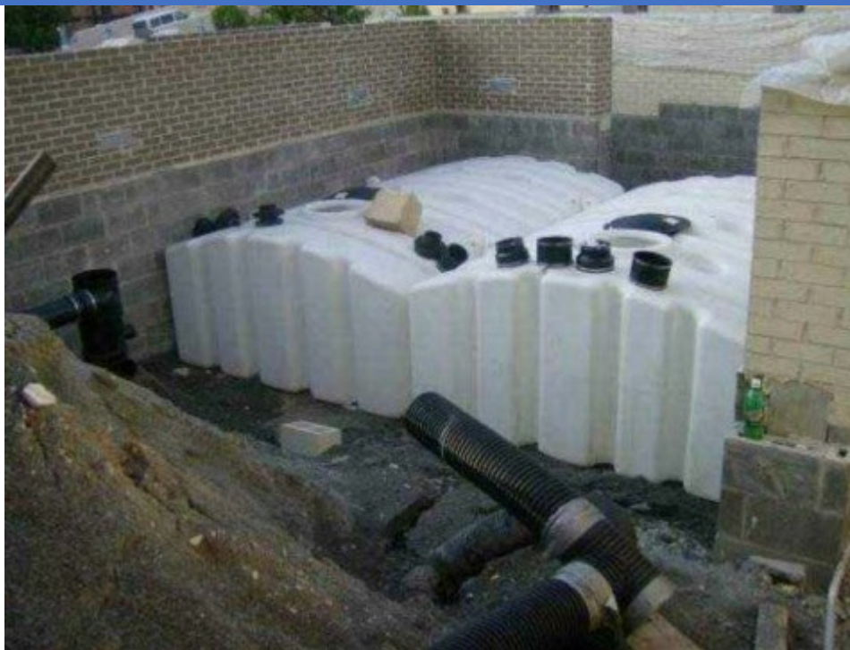
Figure P-BAS-04-5 Example of two Polyethylene Cisterns
