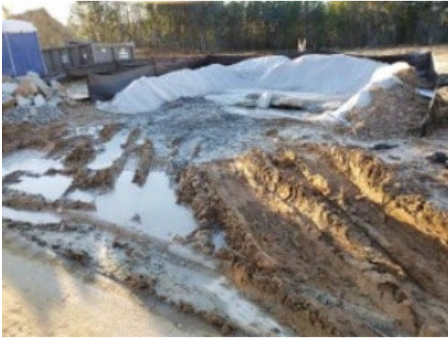
Poorly Maintained Concrete Washout Station
