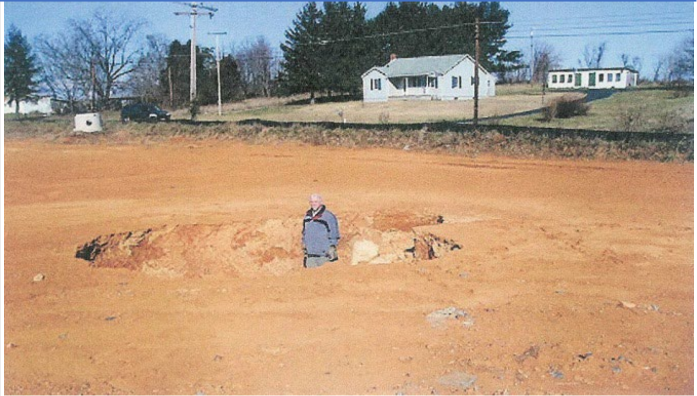
Figure E-18 Sinkhole at a construction site
