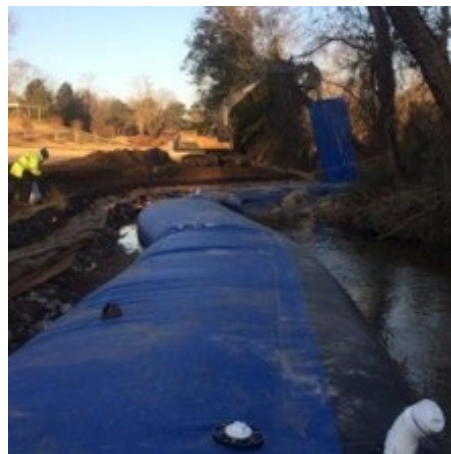
Inflatable Bladder Cofferdam Crossing Source: Detroit Tarp
