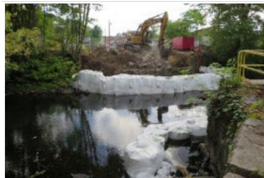
Active Cofferdam Utility Stream Crossing
