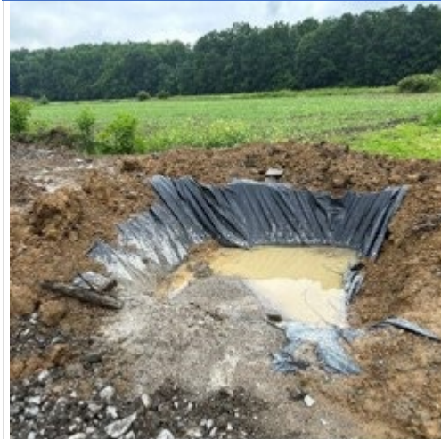
Figure 9-1 Washout Example
