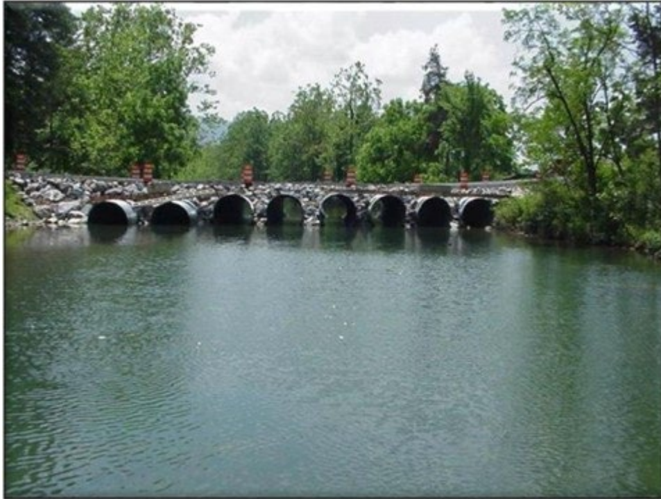
Figure 5-18 Temporary Stream Crossing
