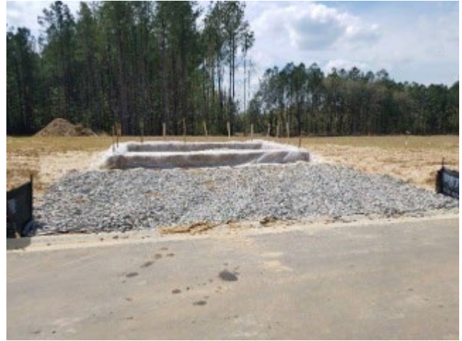
Properly Installed and maintained Concrete Washout Station
