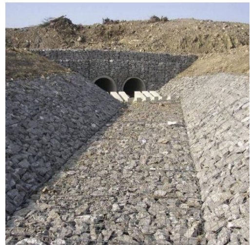
Trapezoidal Gabion Basket Installation Under Dry Conditions
