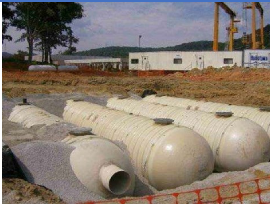
Figure P-BAS-04-4 Example of Multiple Fiberglass Cisterns in Series
