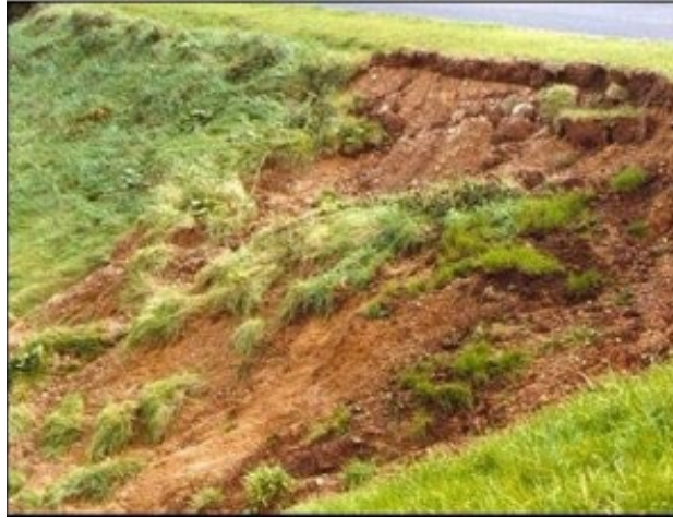
Figure 5-16 Slope Failure from Water Seep
