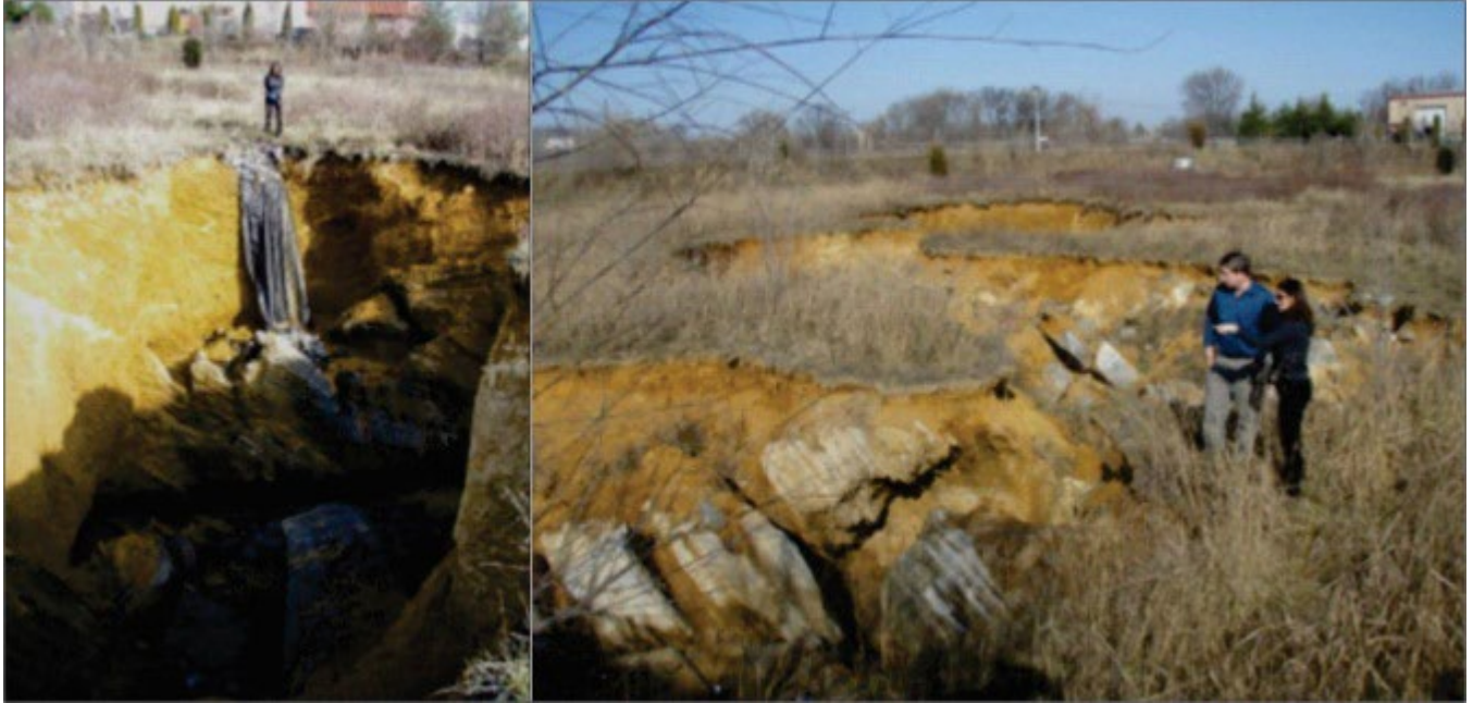
Figure E-9 Subsidence along stormwater conveyance channels
