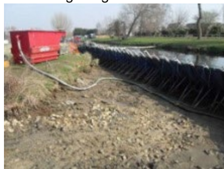
Inflatable Bladder Cofferdam Crossing
