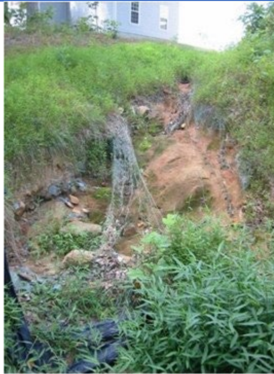
Figure 10-1 An Unmaintained Stormwater Conveyance Channel Generating Sediment to the Receiving Channel
