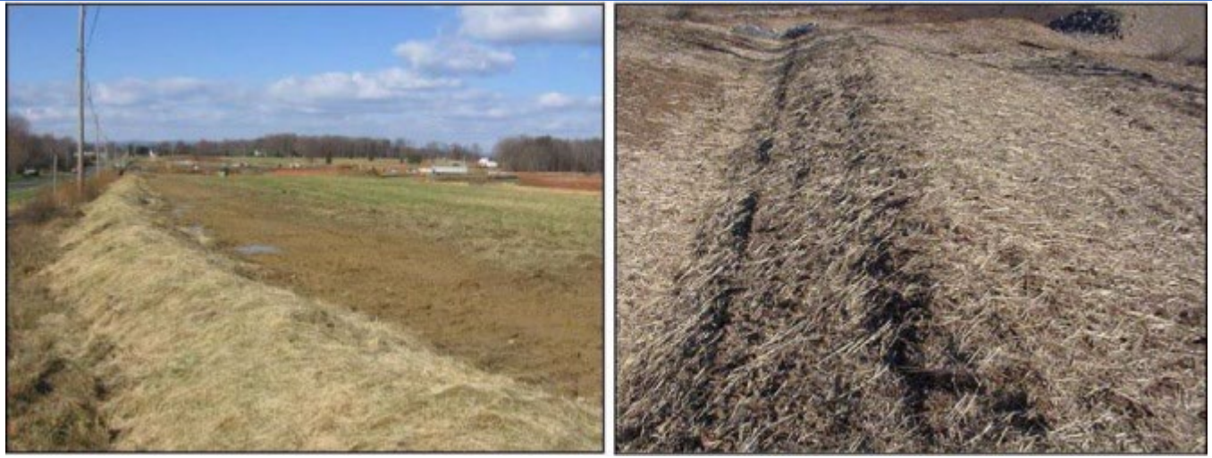
Figure 5-11 Earthen Diversion Structures Seeded and Mulched Immediately After Construction
