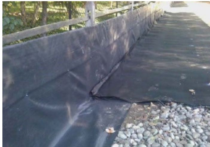
Trenchless Super Silt Fence Installation Source: The Davey Resource Group
