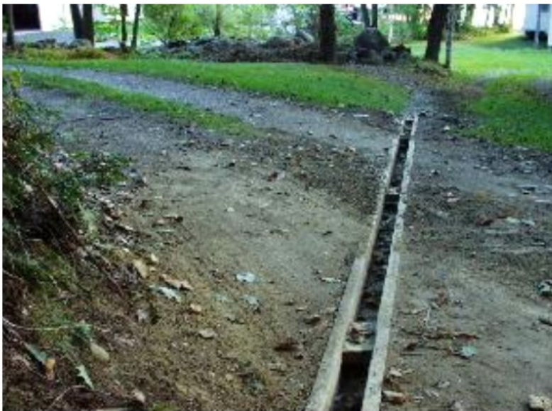
Figure C-ECM-08-4 An open-top culvert along a low-volume driveway
