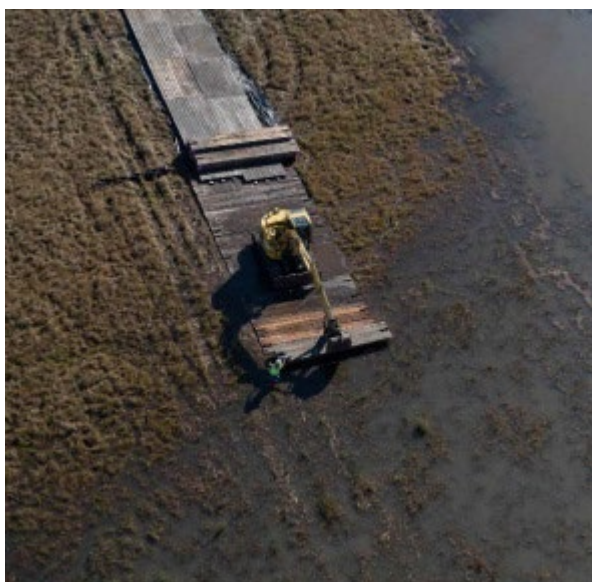
Active Installation of Wooden Wetland Crossing Source: Quality Mat Company 2023
