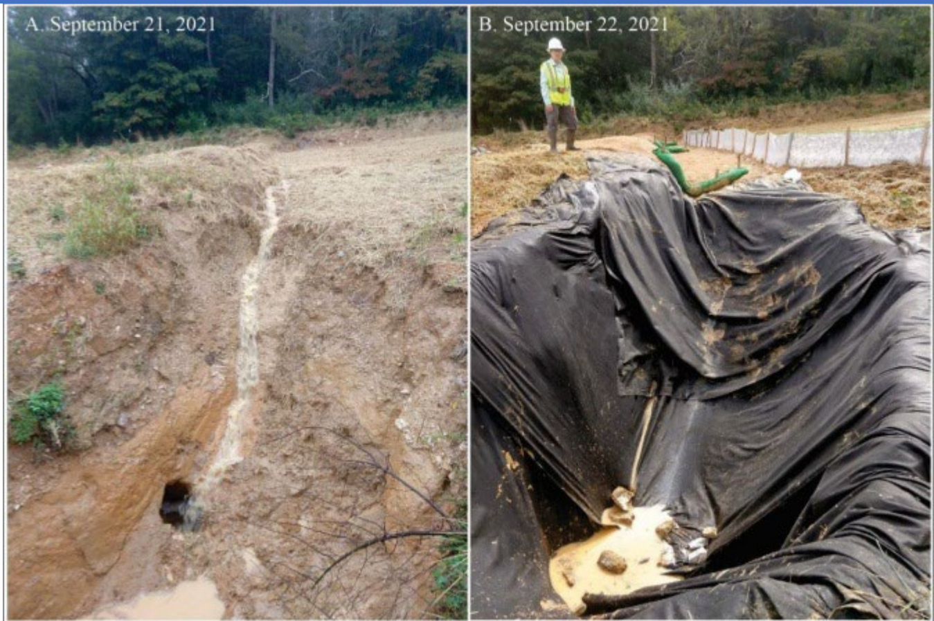
Left: Swallet formed by collapse in sump at end of water bar. Right: same feature, next day after mitigation.
