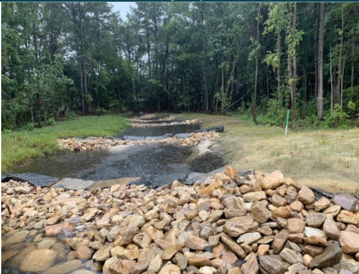
Figure P-CNV-04-1 Newly constructed regenerative stormwater conveyance Chesterfield County Complex
