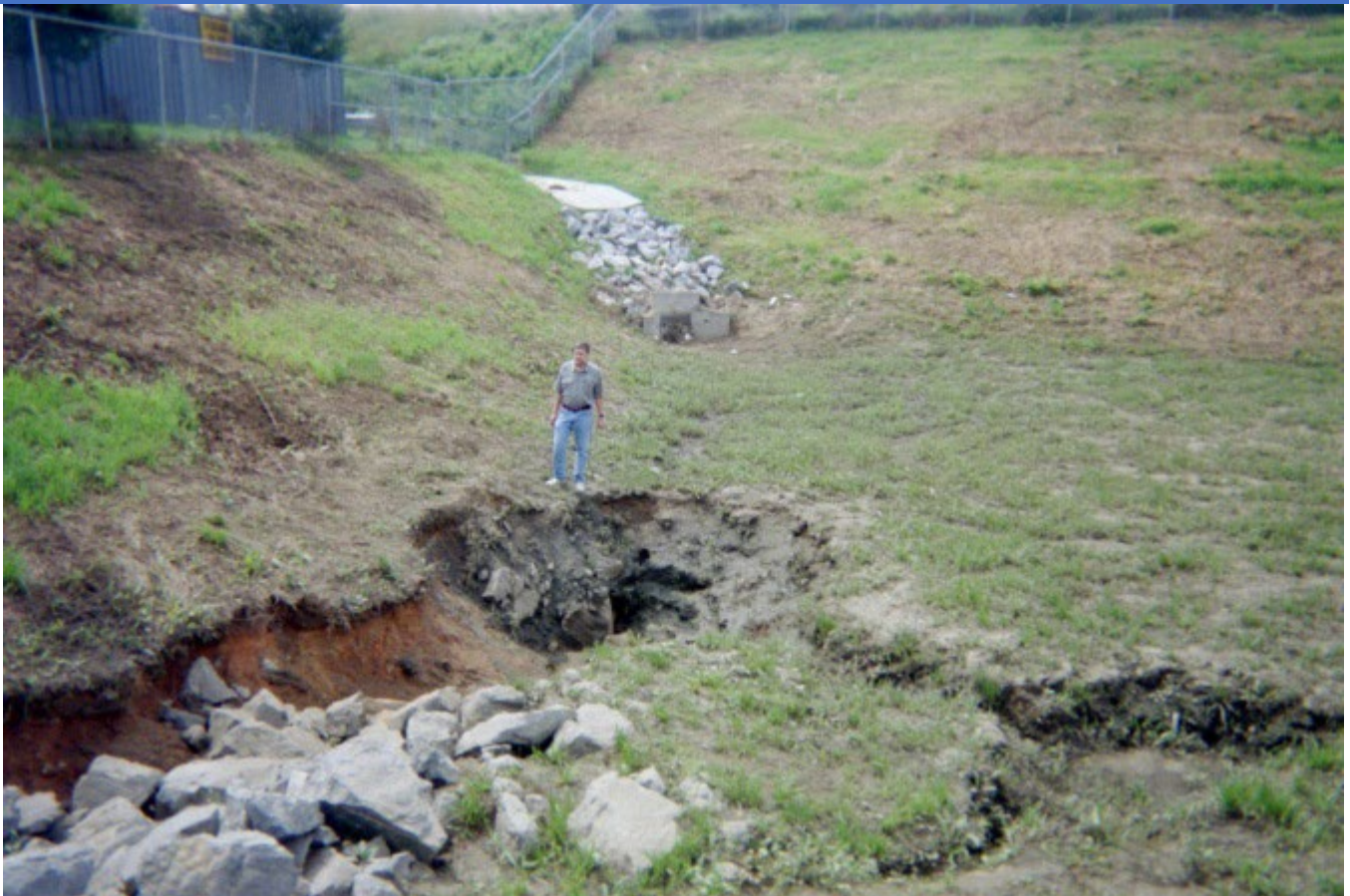
Figure E-10 Typical subsidence failure (sinkhole formation) within a large stormwater detention basin
