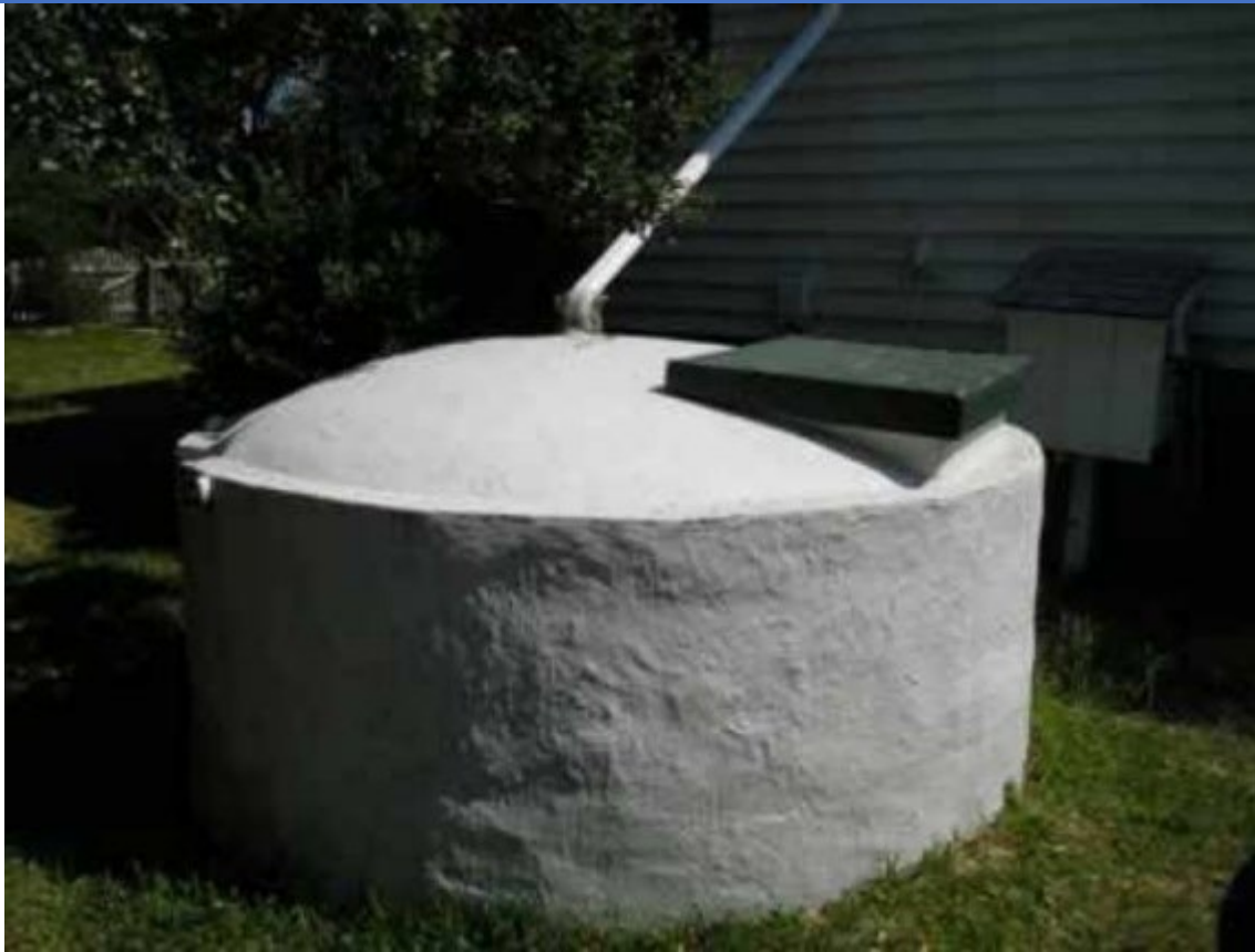
Figure P-BAS- 04-7 Residential Application of a Brick and Stucco Cistern
