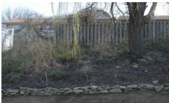
Improperly Installed Compost Blanket on Steep Slope Source: ?
