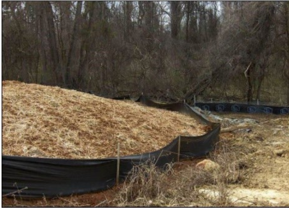
Figure 5-7 Mulch on Stockpile and Protected with Silt Fence
