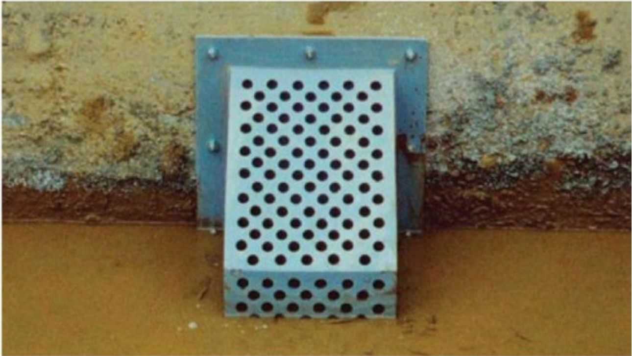
Figure P-SUP-06-5 Manufactured Coarse Solids Screen
