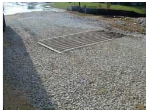
Stone Construction Entrance with Washrack
