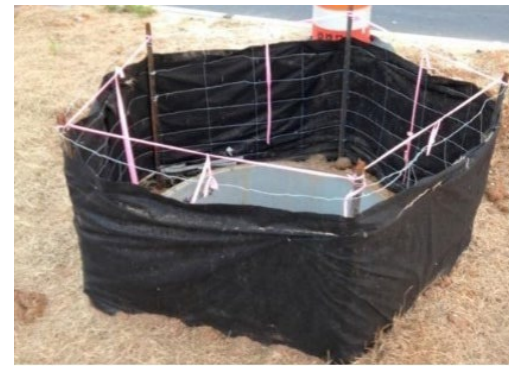
Properly Installed Inlet Protection
