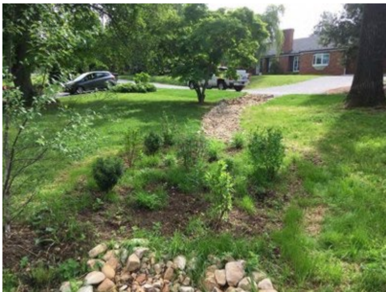
A residential bioretention used to manage upgradient street runoff that was formerly causing nuisance flooding downstream
