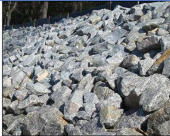
Figure 5-17 Riprap Installation Against Failure
