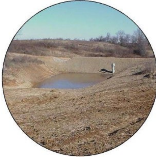
Figure 5-13 Sediment Basin (for drainage area > 3 acres)
