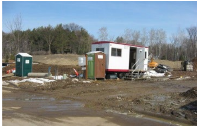
Example of Poorly Maintained Vehicular Route Stabilization
