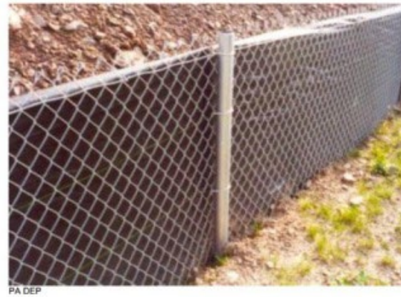
Super Silt Fence Source: PADEP 2012, p.82
