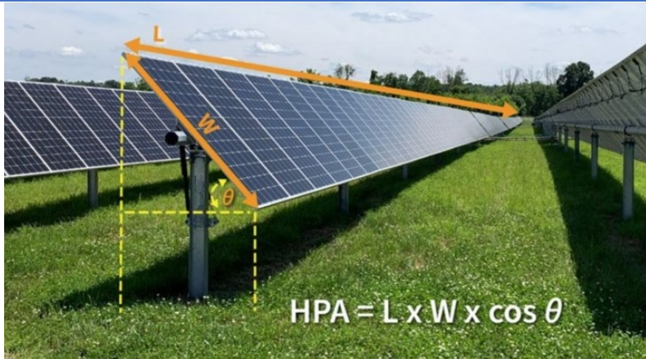
Figure 6-23 Example of Solar Power Array and HPA Calculation Formula
