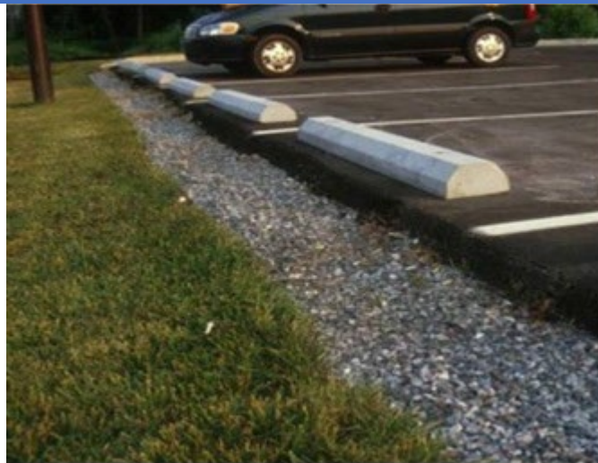
Figure 6-18 Parking Lot Runoff Connected to a Gravel Filter Strip and Grassed Area
