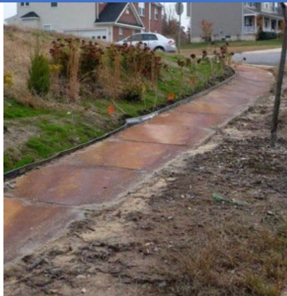
Figure 6-3 Site-Specific Impacts of Acid Sulfate Soil Formation in Construction Fill Materials in Fredericksburg, Virginia
