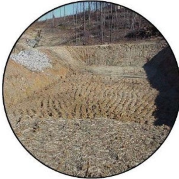
Figure 5-12 Sediment Trap (for < 3 acres)
