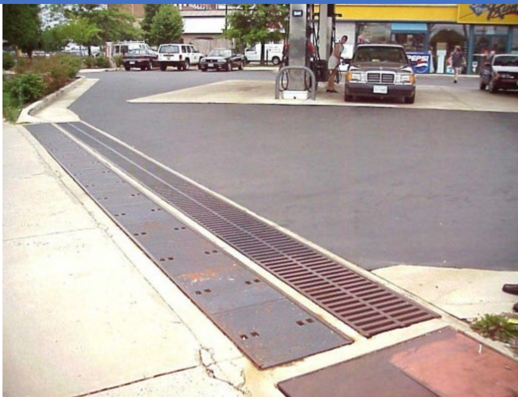
Figure P-FIL-06-3 Perimeter Sand Filter
