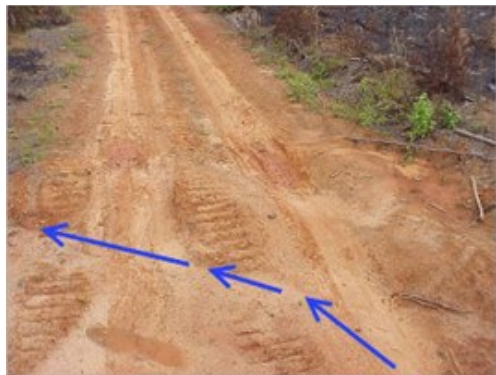
Flow Path along a Right of Way Diversion. Source: Texas A&M Forest Service
