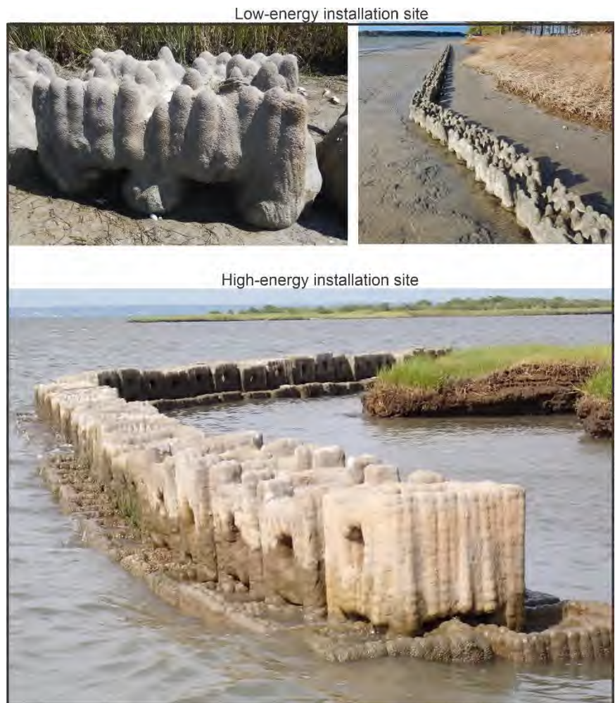
Figure 4-4. Several configurations of 3D printed Natrx modules used at low and high energy sites.
