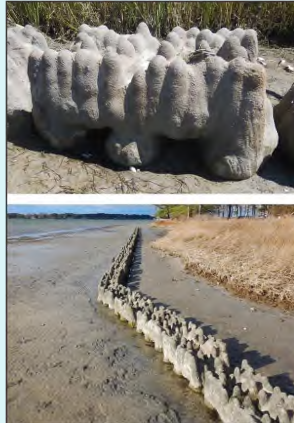
An example of a 3D-printed Natrx living shoreline implemented at another site in Chesapeake Bay.
