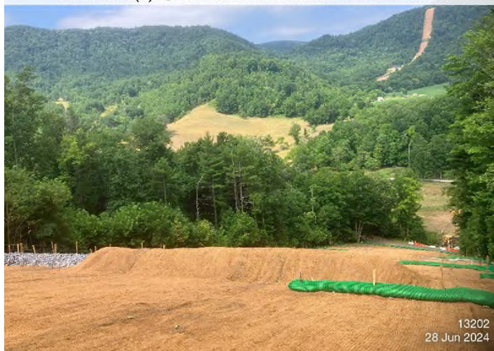
Figure 4: STA 13202+00 – Controls in place and functioning properly.
