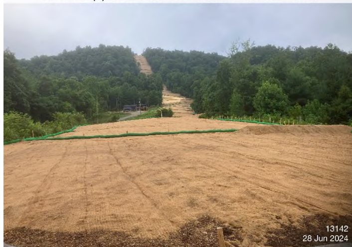
Figure 3: STA 13202+00 – Controls in place and functioning properly.
