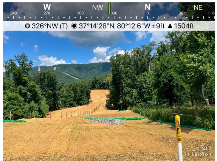
Figure 4: Sta 12400, ESC and permanent waterbars are in place.
