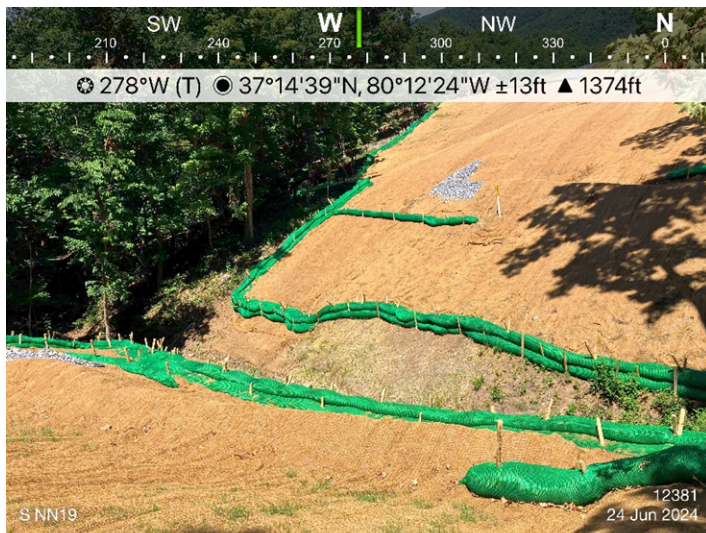
Figure 3: Designated crossing S-NN19, ESC's devices and permanent waterbars are in place.
