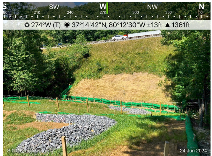
Figure 2: Designated Crossings S-0016, ESC's devices and permanent waterbars are in place.
