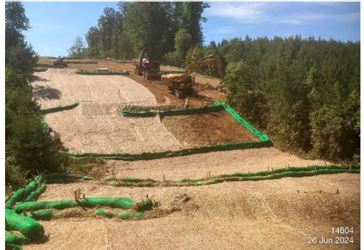
Figure 4: STA 14804+00 – Controls in place and functioning properly.
