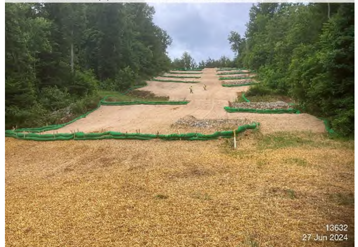
Figure 4: STA 13632+00 – Controls in place and functioning properly.
