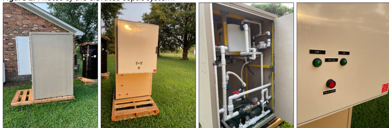
Figure 2. Photos of the elevated septic system.
