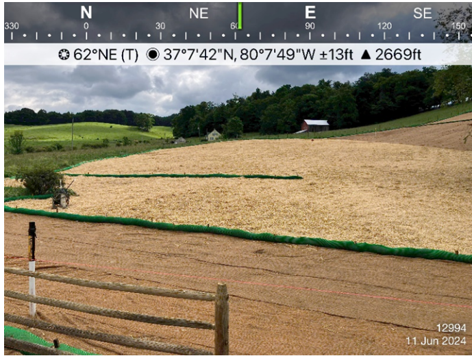
Figure 1: Sta 12994, ESC's devices in place.
