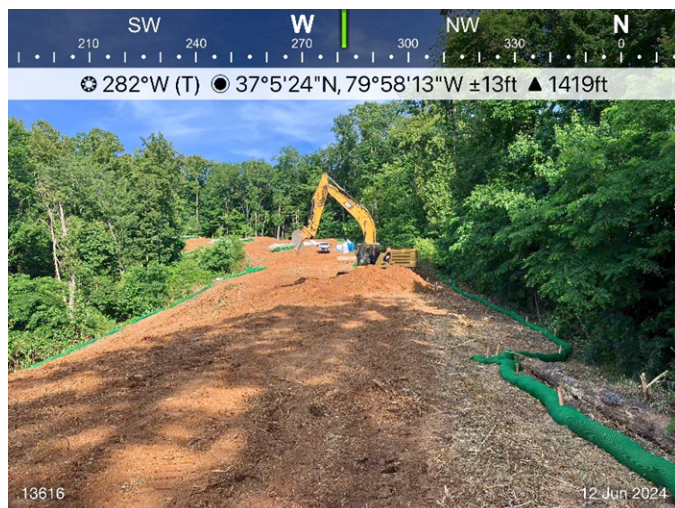
Figure 3: Sta 13613, ESC is in place for active construction.
