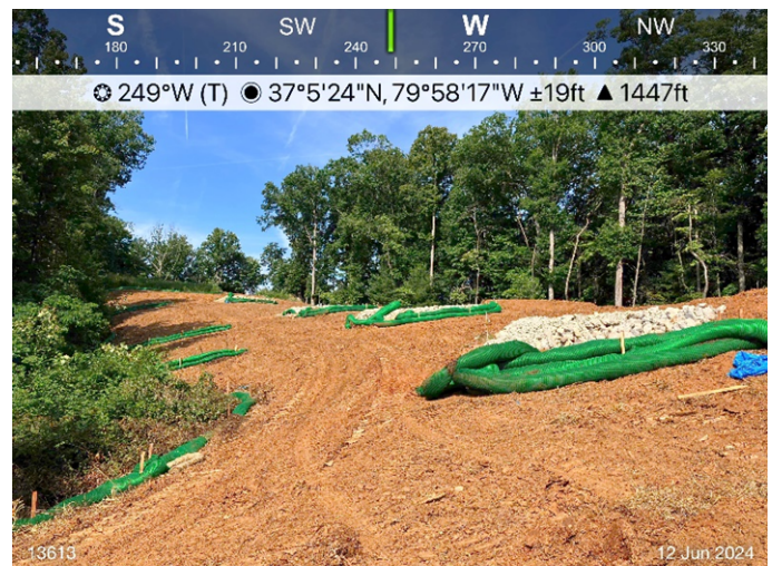
Figure 4: Sta 13613, ESC is in place for active construction.
