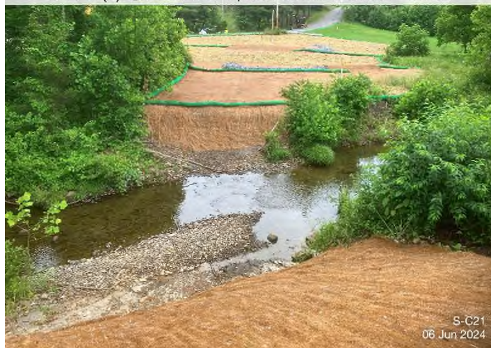
Figure 3: Stream S-C21 – Controls in place and functioning properly.
