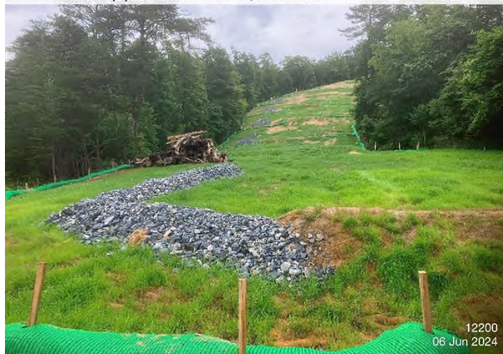
Figure 3: Stream S-C21 – Controls in place and functioning properly.
