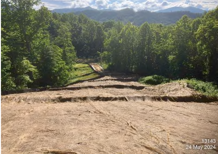
Figure 3: STA 13134+00 – Controls in place and functioning properly.
