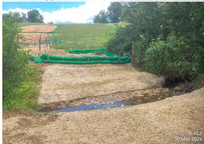
Figure 4: STA 13533+00 – Restabilize denuded area at final grade.
