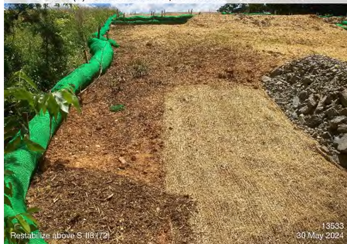
Figure 4: STA 13533+00 – Restabilize denuded area at final grade.
