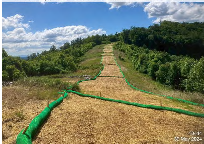
Figure 3: STA 13519+50 – Restabilize denuded area at final grade.
