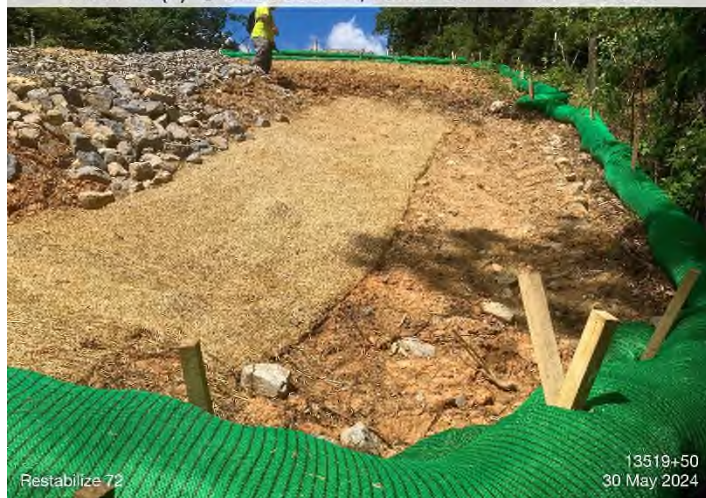
Figure 3: STA 13519+50 – Restabilize denuded area at final grade.
