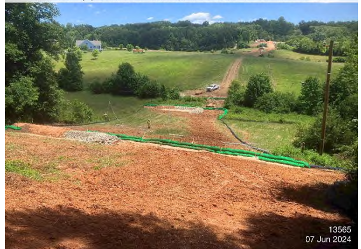
Figure 4: STA 13565+00 – Controls in place and functioning properly. Area actively undergoing final stabilization.
