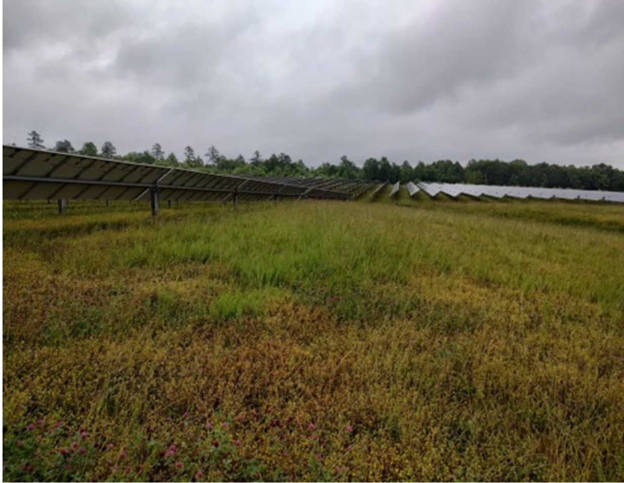
Figure 2. Fully stabilized three-year-old site on a similar Piedmont soil landscape to Figure 1. Once permanently revegetated, sediment losses and stormwater runoff are greatly reduced, but the landscape will still have been considerably transformed with respect to overall landform, soil, and hydrologic conditions. Removal of USS infrastructure at site decommissioning (not shown) will lead to another cycle of soil disturbance that will require some level of remediation, particularly if the land is intended to be returned to pre-existing agriculture or forestry land uses.
